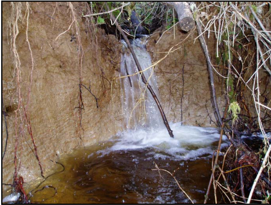
Figure 25. Piling Creek step-pool feature downstream of 2100 Road.
