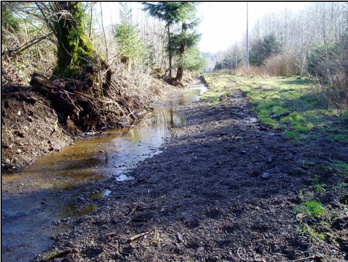
Figure 53. Lost Creek looking upstream at channel diverted by the 2100 Road ditch (noted that ditch is aggraded with sediment and stream was recently flowing across the road).
