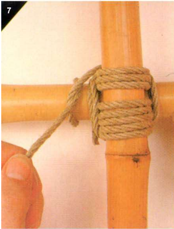
STEP SEVEN. MAKE A CLOVE HITCH AROUND THE HORIZONTAL POLE.
