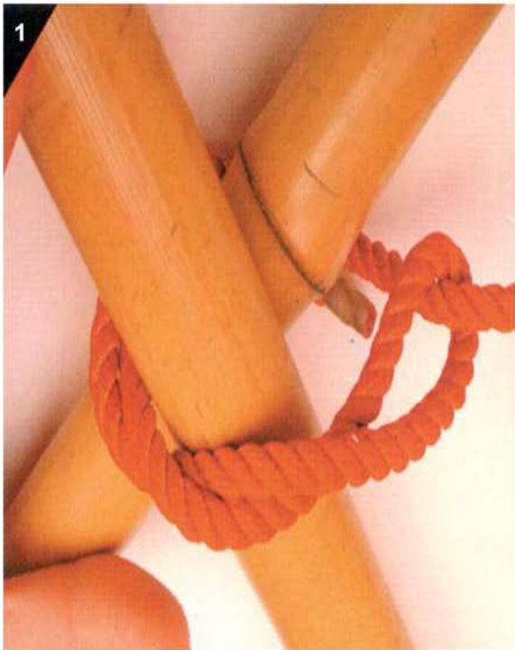
STEP ONE. MAKE A TIMBER HITCH AROUND THE TWO CROSSED POLES.
