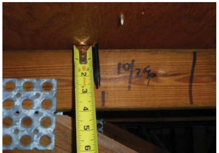
#3 ROOF DECK ATTACHMENT 8d NAILS
