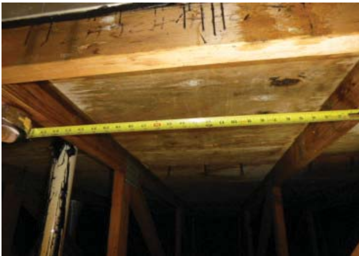
TRUSS/RAFTER SPACING
