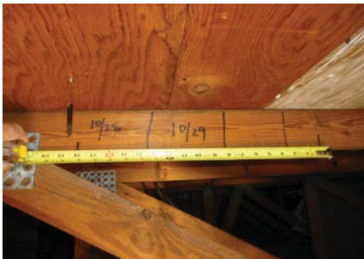
#3 ROOF DECK ATTACHMENT 6" X 6" NAIL SPACING
