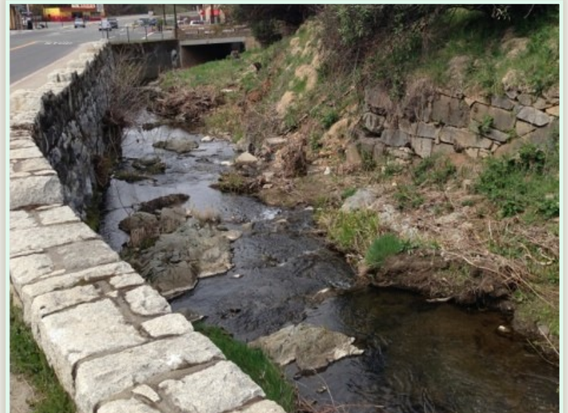
Hangtown Creek at US 50 between Canal Street & Spring Street
