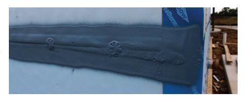
Proceed to flash board joints, penetrations and/or fenestration openings as detailed by the project drawings by spray applying LIQUIDARMOR™ - CM Flashing and Sealant at 50 ±5 wet mils in these areas. A popular technique to attain 50 ±5 wet mils is to apply the product in two passes. This is not required, though, and the target application thickness can be attained in one pass.
