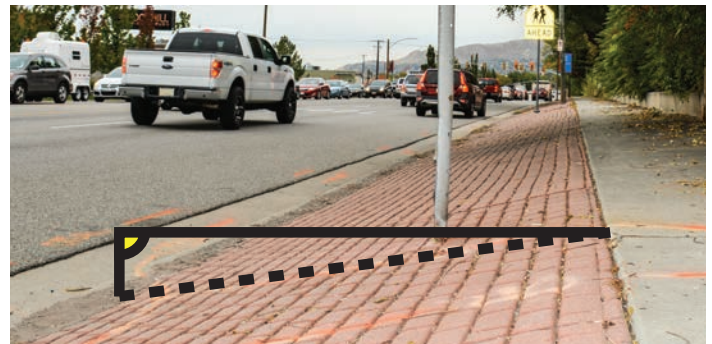
Foothill Drive has a number of narrow sidewalks with significant park strip slopes toward the street which present safety hazards for pedestrians and users with disabilities.
