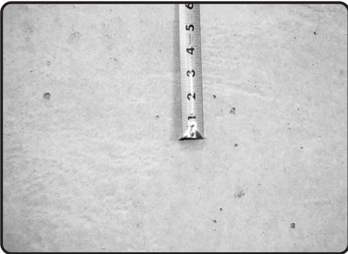
■ **Causes.** Main cause is placement methods. Air is entrapped within the plastic concrete during mixing and placing. Large voids quickly exit the surface. Medium size voids exit during consolidation. Smaller voids are not worked out as easy, tend to stay within the concrete. External vibration will often cause bubbles to collect on the form face. Some form release agents also cause air to collect on the surface.
