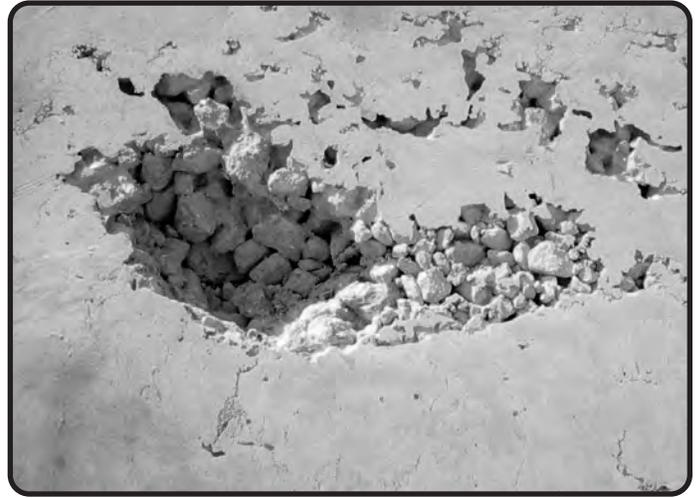
■ **Causes.** Most often caused by improper consolidation, or leaky forms which allows mortar to escape. May also be caused by a stiff, unworkable mix, which cannot be properly consolidated. Coarse aggregate may also separate from mix when dropped from bucket or pump. This separated stone is then pushed into a corner or collects along some obstruction causing a honeycomb.
