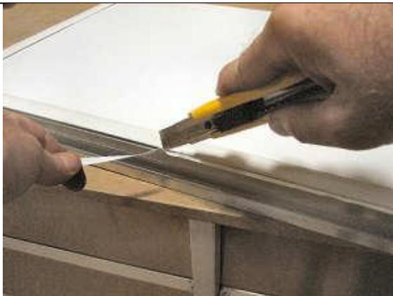
Once the PVC inserts are inserted all around the frame you can remove the extra bleed.
