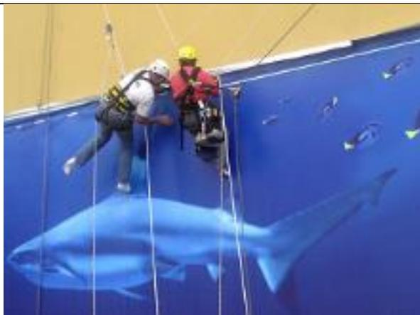
Here you can see the installers replacing the segments (On the left on the photo) by long white PVC inserts (White is recommended for outdoor)
