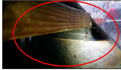
12.5 Item 2(Picture) Fire charred wood supporting stair treads
