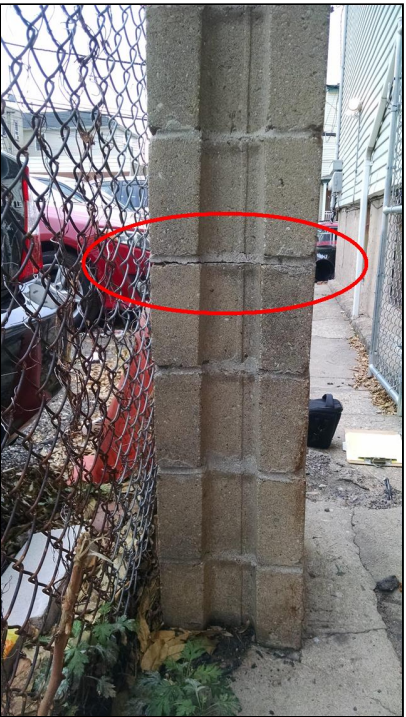
4.1 Item 3(Picture) Crack in mortar joint
