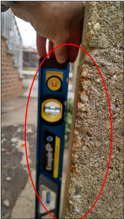
4.1 Item 2(Picture) Bottom of column not plumb
