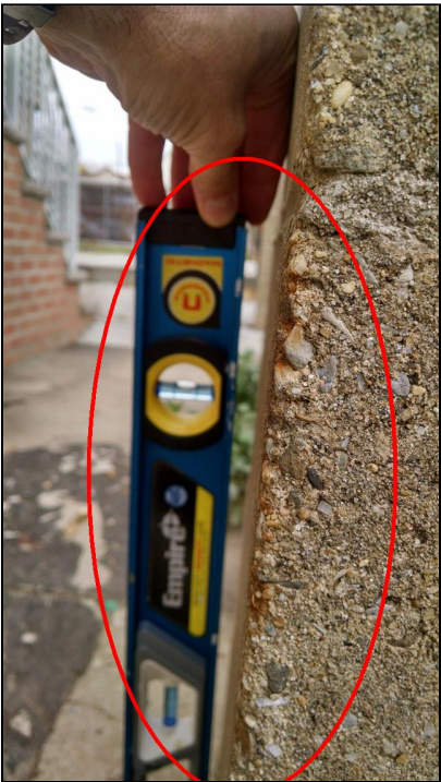
4.1 Item 2(Picture) Bottom of column not plumb
