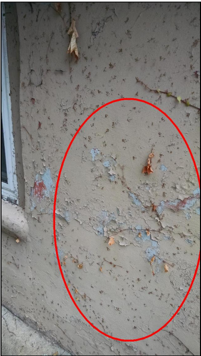
4.0 Item 8(Picture) Peeling paint left side
