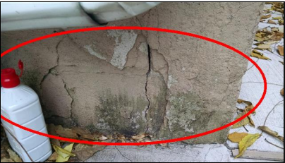
4.0 Item 6(Picture) Parging cracked in rear
