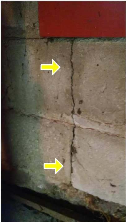
4.0 Item 17(Picture) Crack-interior right side basement wall
