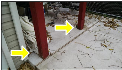
2.8 Item 20(Picture) No mechanical connectors
