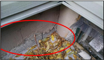
4.0 Item 11(Picture) Parging deteriorated in rear
