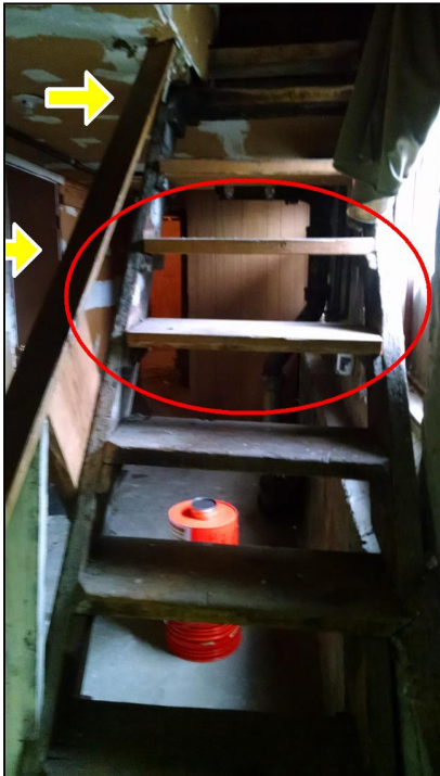
12.5 Item 1(Picture) Open risers, handrail too low and no balusters
