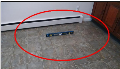
4.5 Item 13(Picture) Hump in 1st floor kitchen floor
