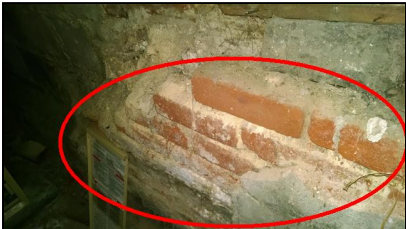
4.0 Item 16(Picture) Brick foundation in rear deteriorated
