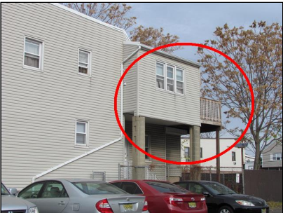
2.8 Item 13(Picture) Deck attached to cantilevered portion of the house
