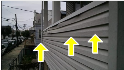
2.0 Item 4(Picture) Vinyl siding buckling on front porch
