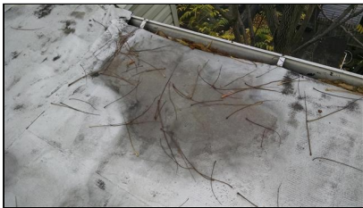
5.0 Item 4(Picture) Ponding water on flat roof
