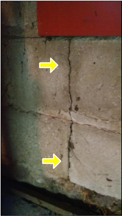
4.0 Item 17(Picture) Crack-interior right side basement wall
