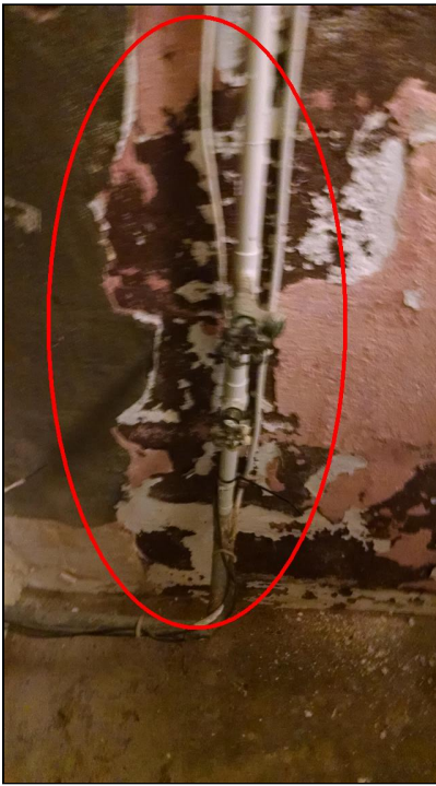
4.0 Item 19(Picture) Peeling paint and parging deteriorated in front basement
