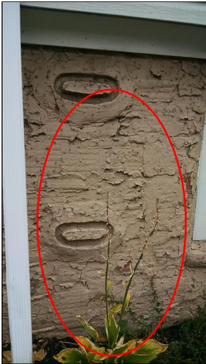
4.0 Item 1(Picture) Peeling paint front
