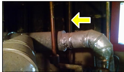
9.1 Item 2(Picture) Vent sloped downward
