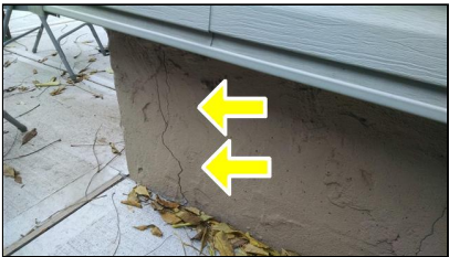
4.0 Item 9(Picture) Cracks in rear
