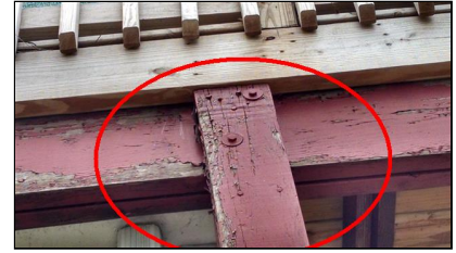
2.8 Item 19(Picture) No mechanical connectors
