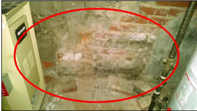
4.0 Item 15(Picture) Brick foundation wall in rear deteriorated- bricks laying on floor
