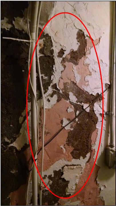
4.0 Item 18(Picture) Peeling paint and parging deteriorated in front basement
