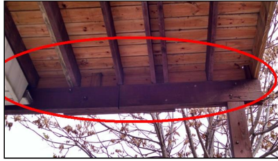
2.8 Item 18(Picture) No joist hangers
