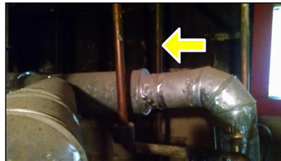
9.1 Item 2(Picture) Vent sloped downward
