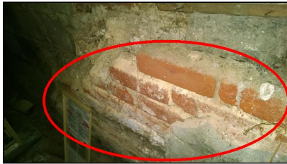
4.0 Item 16(Picture) Brick foundation in rear deteriorated
