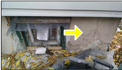
4.0 Item 10(Picture) Cracks in rear
