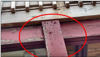
2.8 Item 19(Picture) No mechanical connectors
