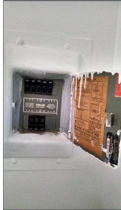
7.4 Item 3(Picture) 1st floor Federal Pacific sub panel
