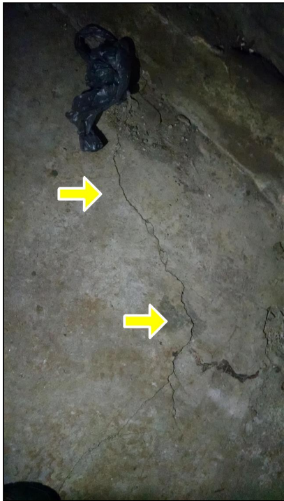
4.0 Item 13(Picture) Cracks in basement floor
