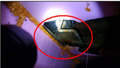
4.5 Item 2(Picture) Charred wood-1st floor bathroom
