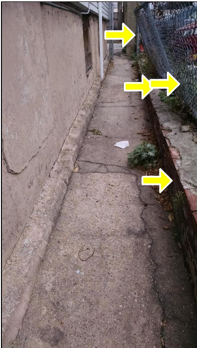
1.5 Item 1(Picture) Right side retaining wall and fencing is in need of repairs
