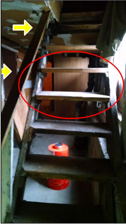
12.5 Item 1(Picture) Open risers, handrail too low and no balusters
