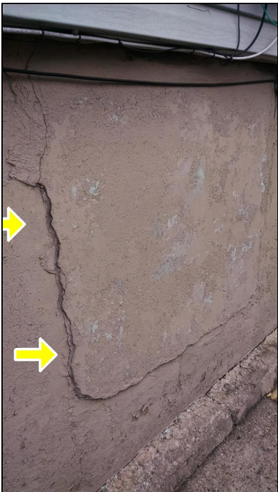
4.0 Item 4(Picture) Cracks on right side
