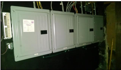
4 electric main service panels in basement
