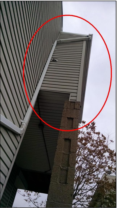
4.1 Item 6(Picture) Columns supporting rear of house
