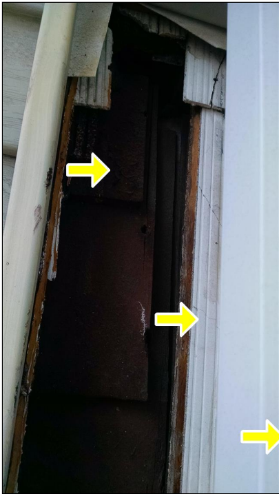
2.0 Item 3(Picture) 3 layers of siding
