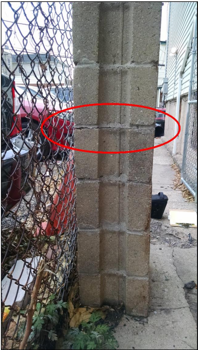
4.1 Item 3(Picture) Crack in mortar joint
