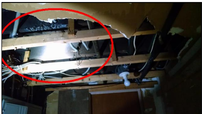
10.0 Item 3(Picture) Charred floor joists in front of basement
