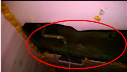
4.5 Item 1(Picture) Charred wood-1st floor bathroom
