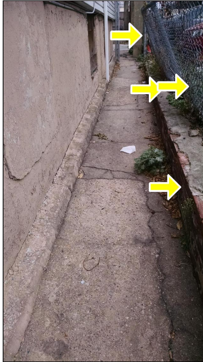
1.5 Item 1(Picture) Right side retaining wall and fencing is in need of repairs
