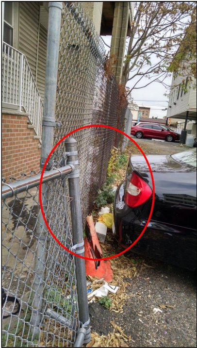
4.1 Item 5(Picture) Columns have no protection from cars parking in the parking lot on the right side of the house
