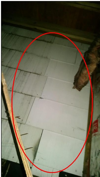
2.0 Item 5(Picture) Fiber cement siding visible in rear basement stairwell
