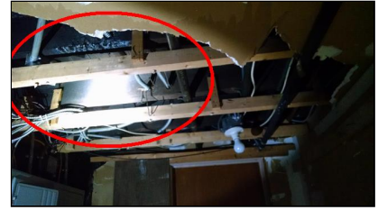
10.0 Item 3(Picture) Charred floor joists in front of basement
