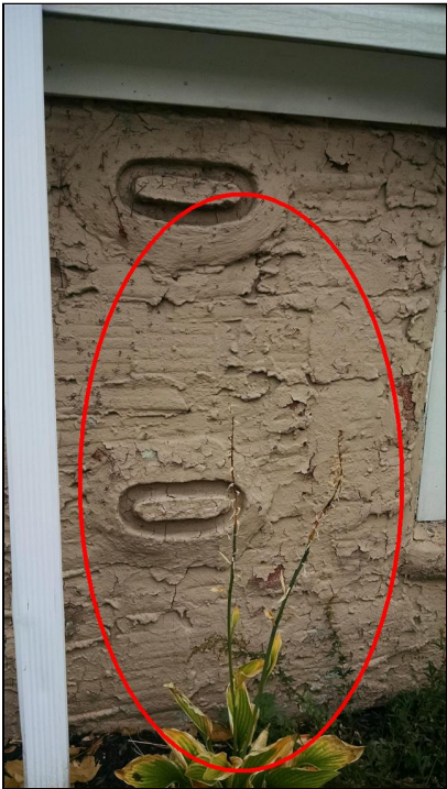
4.0 Item 1(Picture) Peeling paint front
