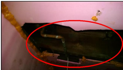
4.5 Item 1(Picture) Charred wood-1st floor bathroom
