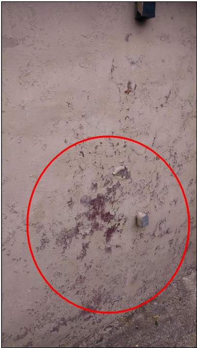
4.0 Item 2(Picture) Peeling paint left side
