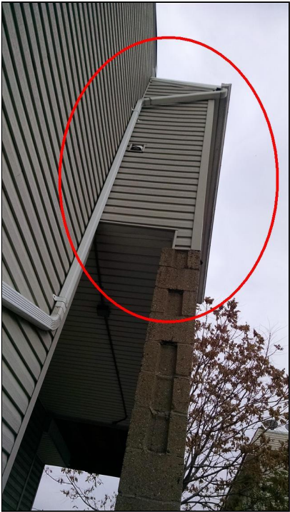
4.1 Item 6(Picture) Columns supporting rear of house
