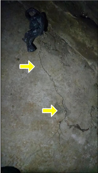
4.0 Item 13(Picture) Cracks in basement floor
