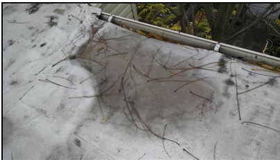
5.0 Item 4(Picture) Ponding water on flat roof
