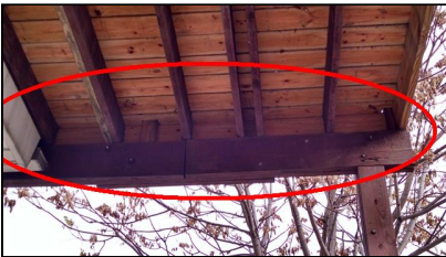
2.8 Item 18(Picture) No joist hangers
