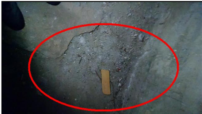
4.0 Item 12(Picture) Cracks in basement floor
