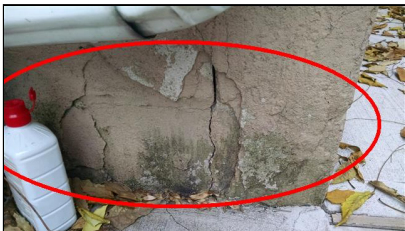
4.0 Item 6(Picture) Parging cracked in rear
