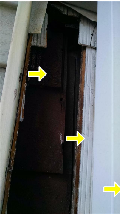
2.0 Item 3(Picture) 3 layers of siding
