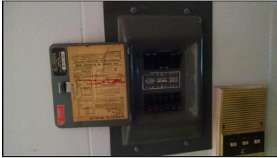
7.4 Item 1(Picture) 2nd floor Federal Pacific sub panel
