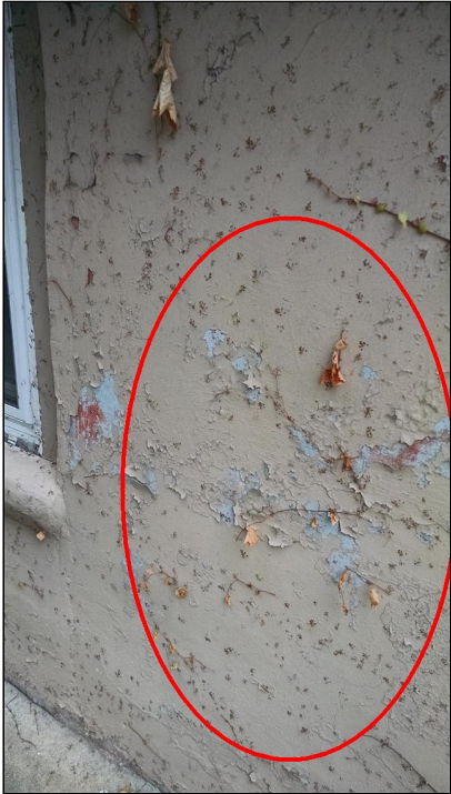
4.0 Item 8(Picture) Peeling paint left side
