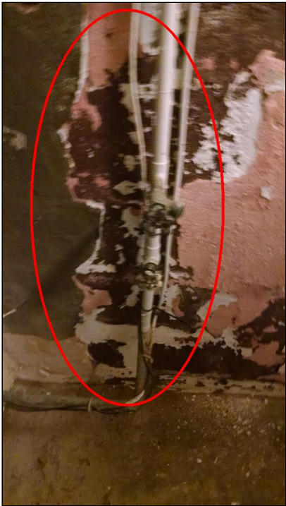
4.0 Item 19(Picture) Peeling paint and parging deteriorated in front basement
