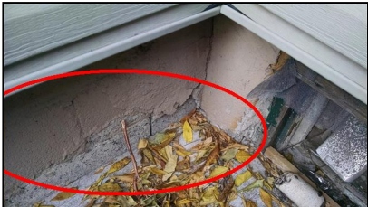
4.0 Item 11(Picture) Parging deteriorated in rear
