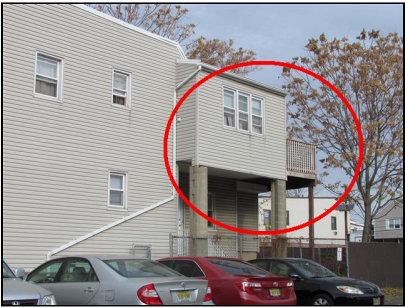
2.8 Item 13(Picture) Deck attached to cantilevered portion of the house
