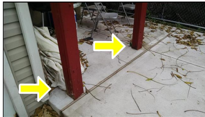
2.8 Item 20(Picture) No mechanical connectors
