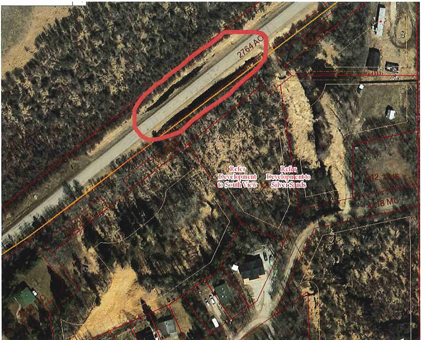
For everyone's reference the area we are talking about is circled in red above. The length of asphalt removal/repair is approximately 100 m long.
