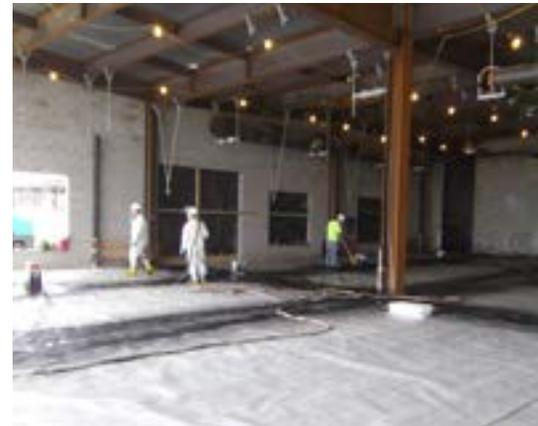
Approved LIQUID BOOT® 500 installer, Environmental Management Specialists, Inc., ensured a proper installation and a vapor-tight seal around all penetration and footings, critical vapor intrusion pathway areas that present the most potential risk for compromised indoor air quality within the structure. LIQUID BOOT® 500 can only be installed by those trained and approved by CETCO, helping to ensure a quality and reliable gas vapor membrane system for your project.
