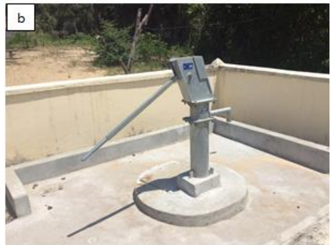
Figure 17: Ampanalana non-operational bucket well (a) and MEN PAUET Indian Pump (b), with well depth of 10.5m, water at 8m and production of 25 liters/min.
