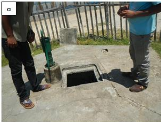
Figure 17: Ampanalana non-operational bucket well (a) and MEN PAUET Indian Pump (b), with well depth of 10.5m, water at 8m and production of 25 liters/min.
