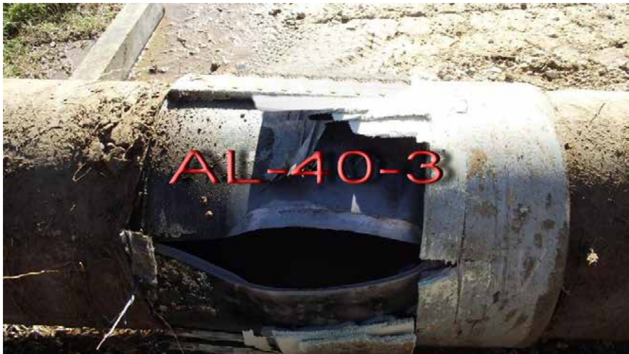
Figure 4 – Photograph of Failure Location, 40% Corrosion Sample
