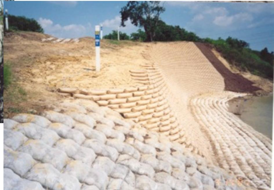
Here we were restricted by the profile of the pipeline. By having the flexibility to combine several different methods, we were able to protect the pipeline and not constrict the drainage flow.
