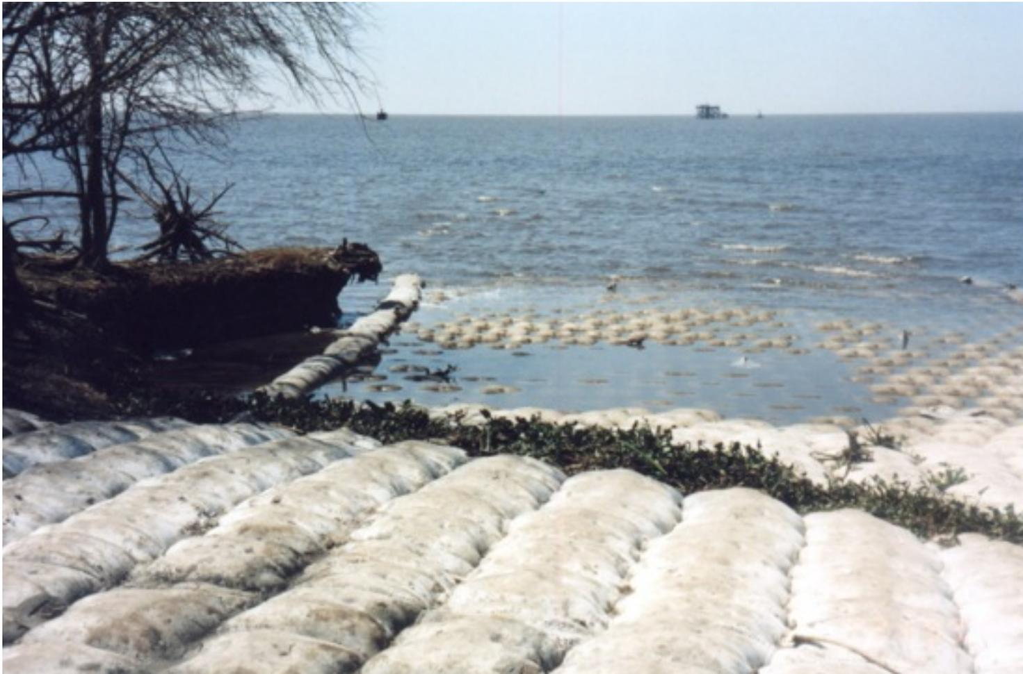
Eco-Flex mats are fabricated using a combination of solid and unfilled elements which allow vegetation growth.
