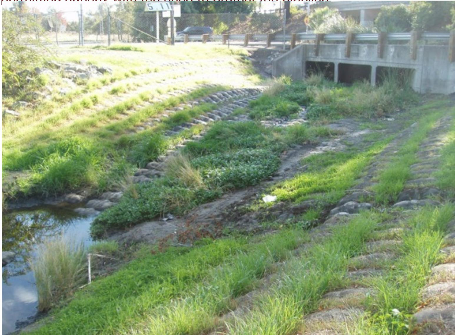
The pipelines are exposed in the foreground. A tremendous volume of water comes through these culverts. The primary concern at this site was the dissipation of energy.
