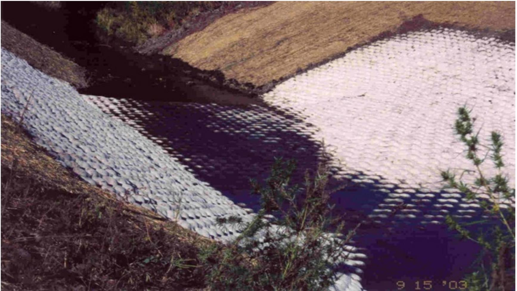
Subsea Pipeline Stabilization. There are characteristics of many open water applications that lend themselves to the use of pre-cast mats. We have used them extensively in the right applications. Due to their inability to accommodate a compound radius, low unit weight, an inferior hydraulic shape and the propensity to under-scour we never use them in rivers or streams that are subject to bank full flow.
