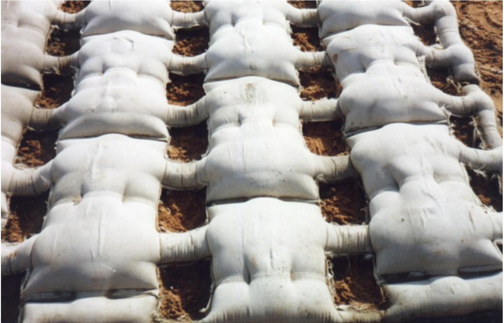
Eco-Flex Mats are identical to Ercoform but include open cells to provide environmentally friendly protection against periodic high flow conditions.
