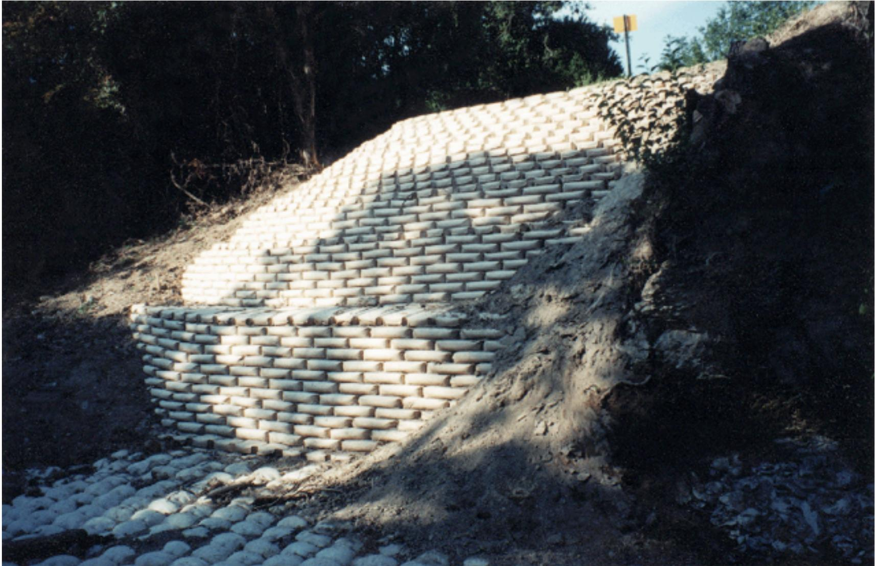
In critical installations, geo-grid material is placed between the field dirt lifts as a high tech method of soil reinforcement. Above each of the geo-grid lining, a 4 inch perforated drain pipe is installed which vents water presence and eliminates the build up of hydrostatic pressure.
