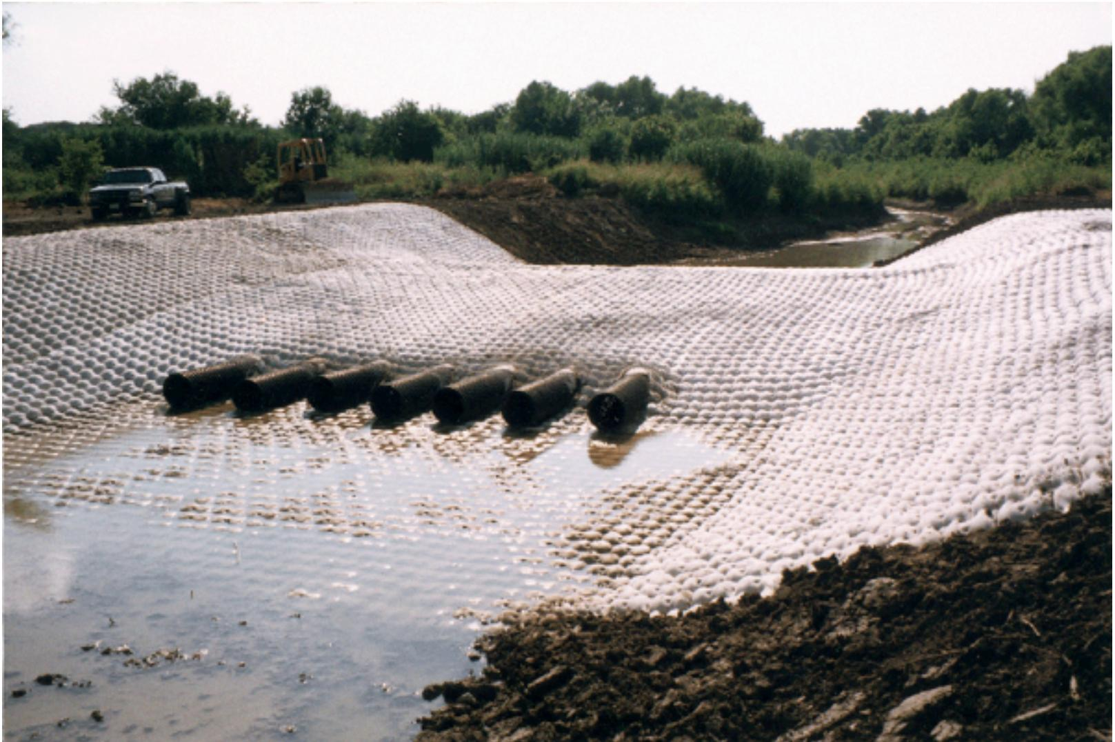
**Grout Mats for Shore Protection:** This beach approach is another example of the flexibility of this system. The pipeline was exposed or had shallow cover to 1000' from the shore. The design had to accommodate the effects of wave energy dissipation, both over the Mat and along the perimeter. It incorporates large cylindrical scour brakes which prevent the mat from being lifted or undermined.
