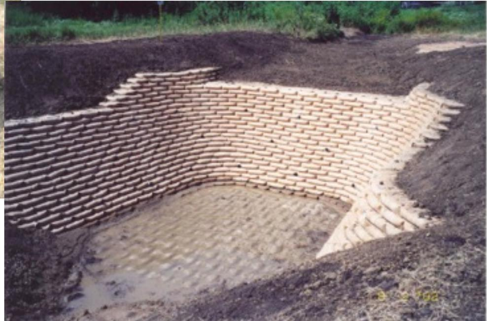
A flexible revetment was used to protect the banks and a Mat was designed to withstand the impact of the vertical drop and the resulting hydraulic jump.
