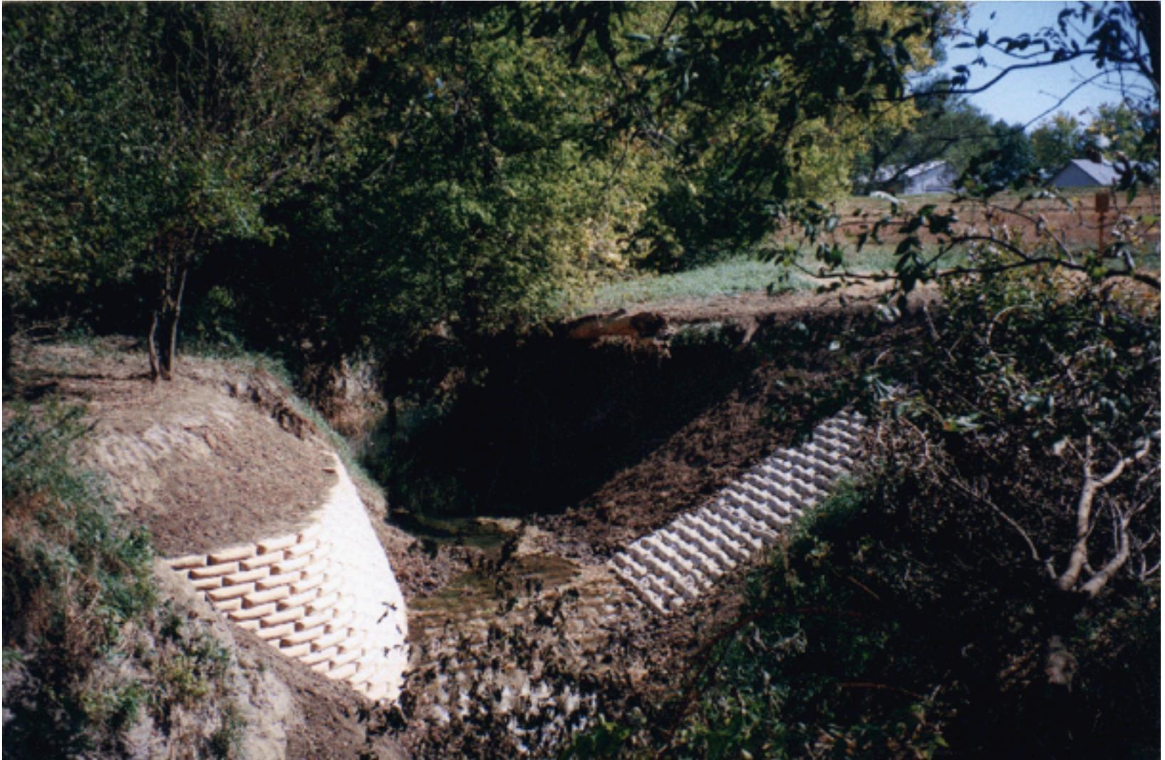
This project required that we conform to the irregular shape of the natural bank and also provide bottom protection.
