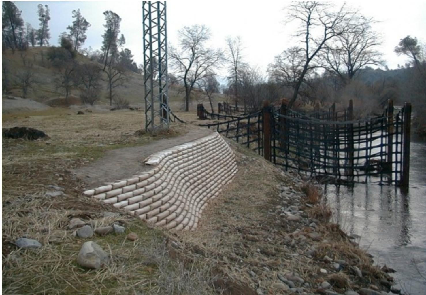
Mats, when filled with grout, form cable reinforced articulating concrete block mattresses that resist erosive forces. This type of mat is normally pumped from the bottom first and then pumped up the ascending slope.
