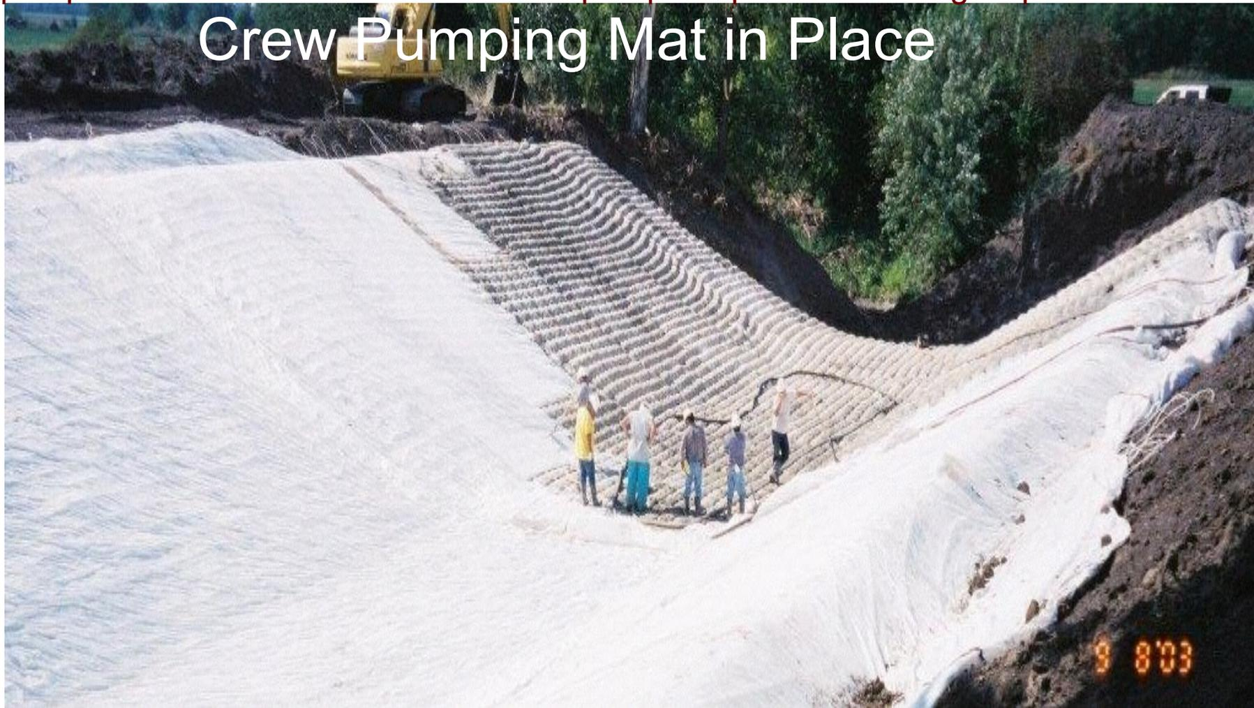
Shows a fully pumped Mat that has been blended with the surrounding environment in a functional manner.
