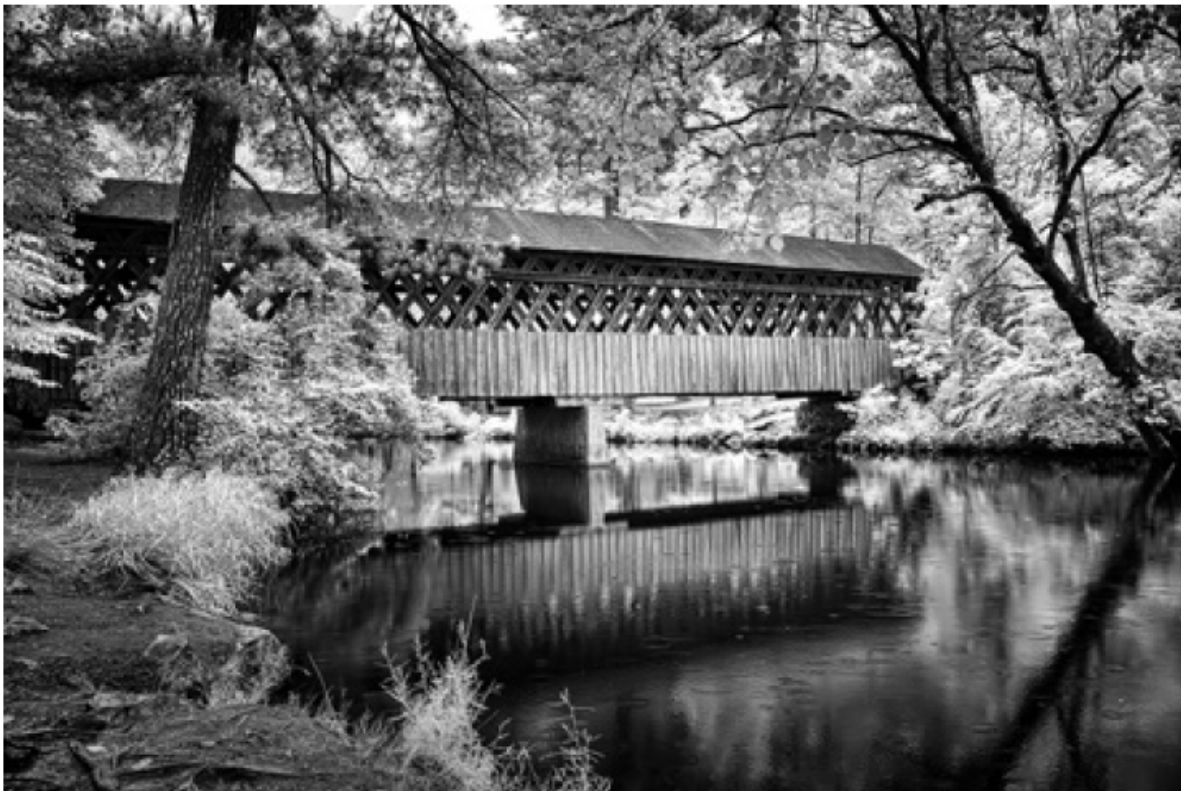
Pooles Mill Bridge
