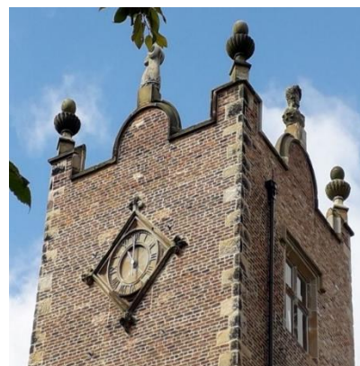
Restored tower top
