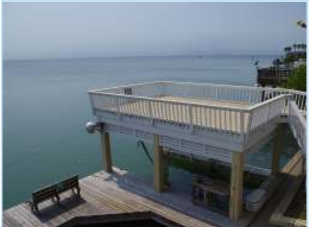
Deck Above Boat Lift
