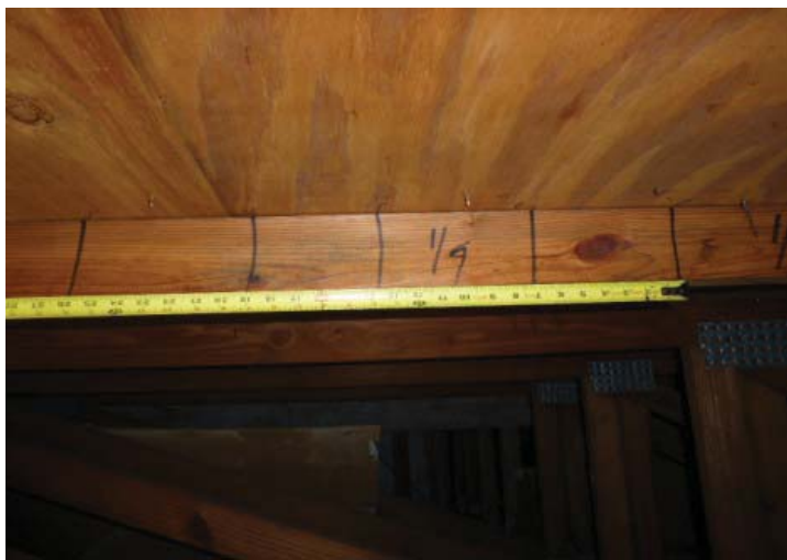
#3 ROOF DECK ATTACHMENT 6" X 6" NAIL SPACING
