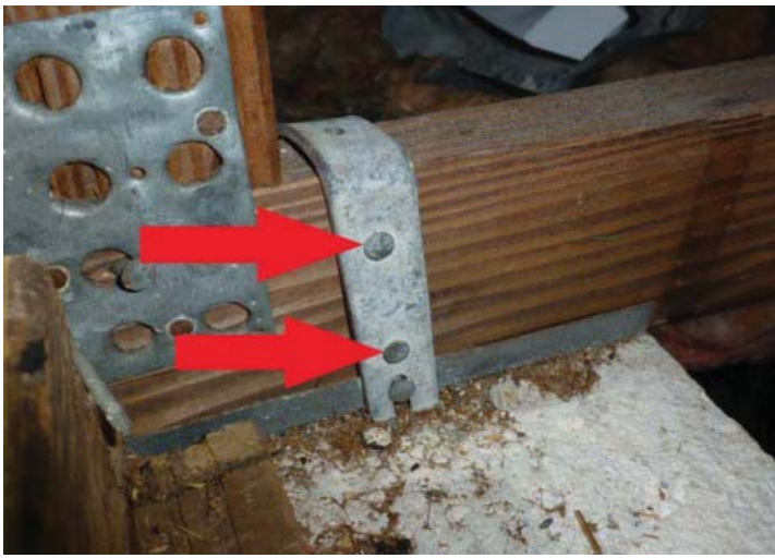
#4 ROOF TO WALL ATTACHMENT FACE SIDE
