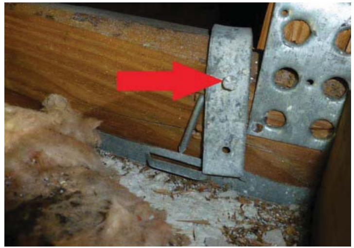
#4 ROOF TO WALL ATTACHMENT OPPOSITE SIDE
