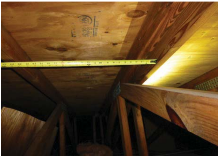
TRUSS/RAFTER SPACING
