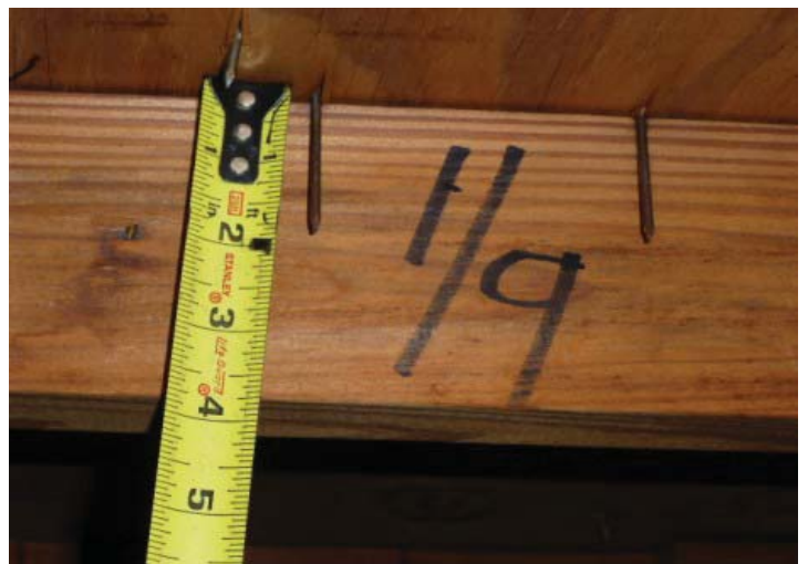
#3 ROOF DECK ATTACHMENT 8d NAILS
