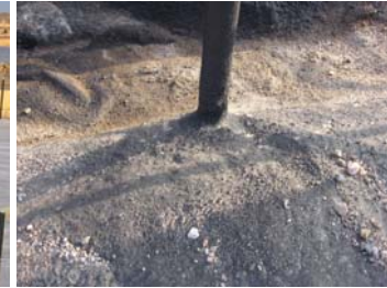
2. Seal barrier directly to VaporStake™
