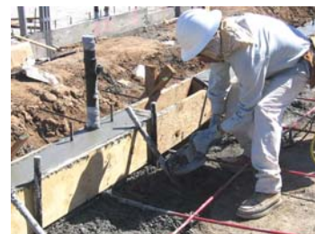
4. Cut VaporStake™ above the seal but below the finished surface
