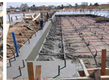
5. Permanently leave the lower portion of VaporStake™
