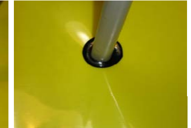
2. Properly align the nail holes and drive the VaporStake™ through the StegoWrap®. The VaporStake™ can be turned while the mastic is wet, but do not turn it after the mastic has set up.
