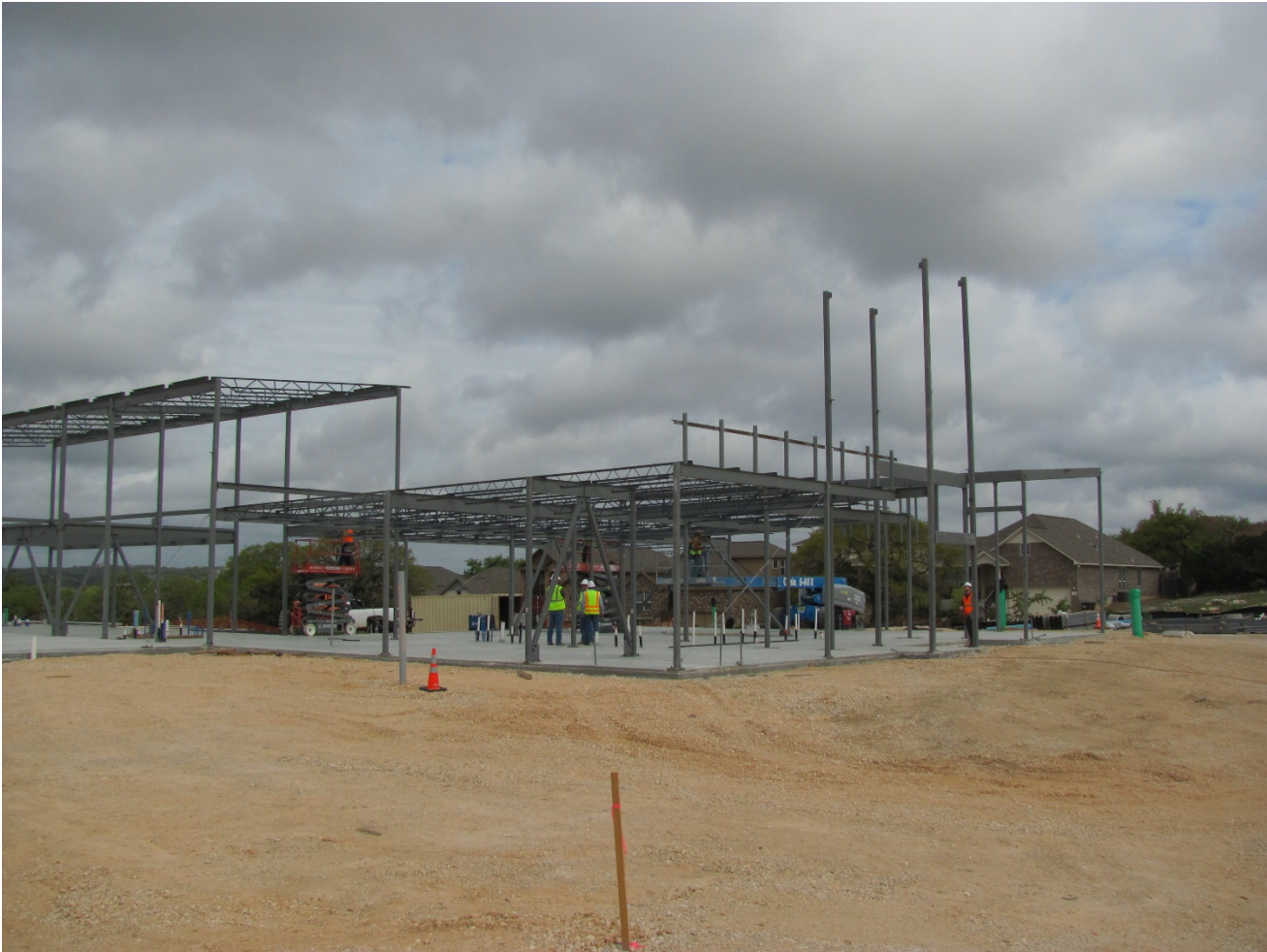
EXHIBIT 9 – STRUTURAL STEEL ERECTION – WORKING DAY 9 04.05.21
