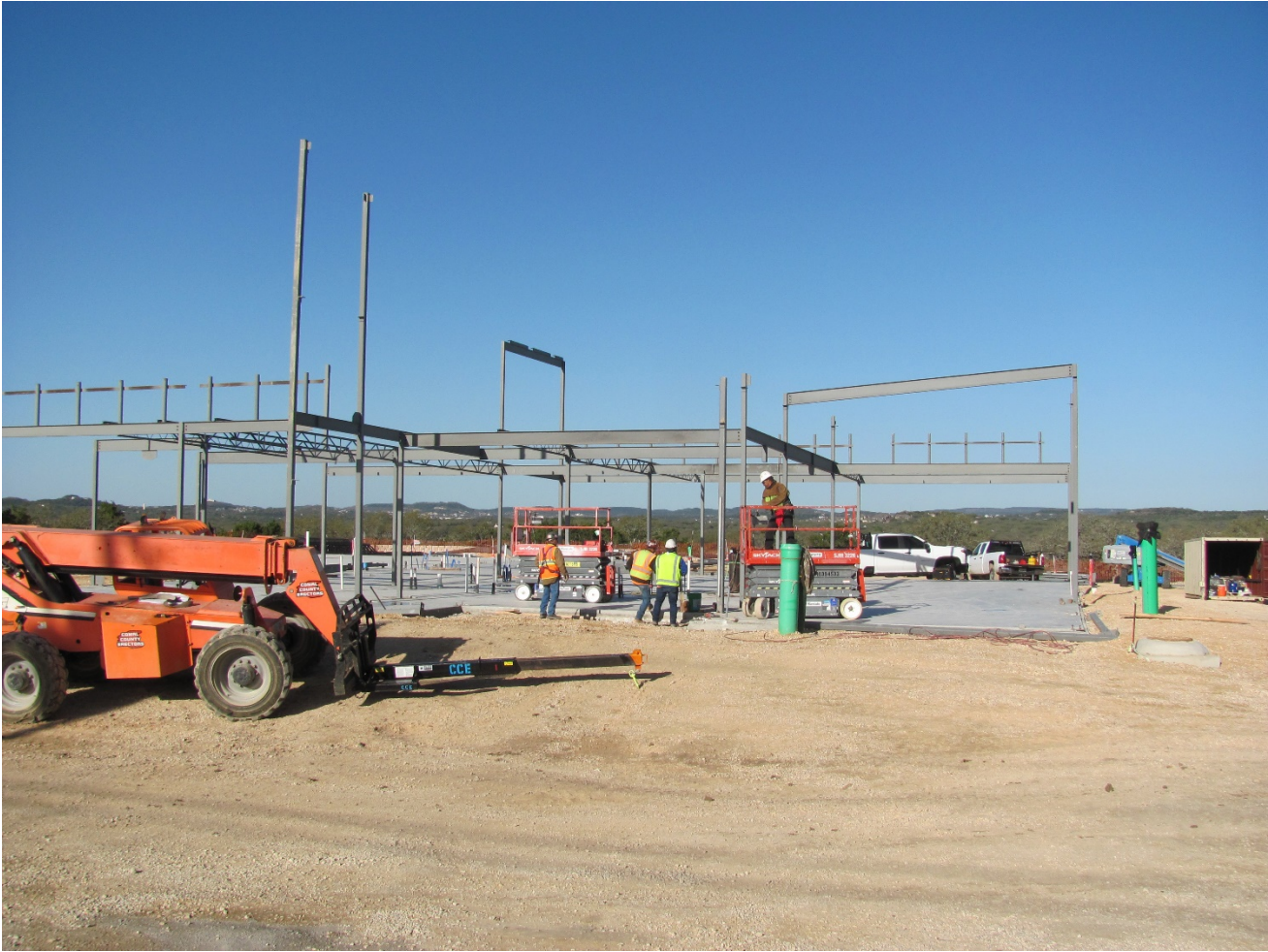
EXHIBIT 4 – STRUCTURAL STEEL ERECTION – WORKING DAY 3 03.25.21
