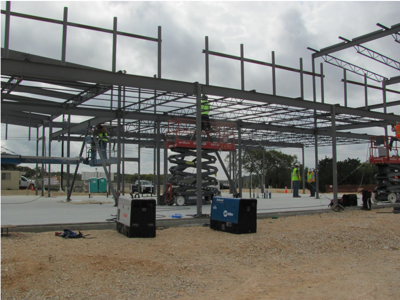
EXHIBIT 8 – STRUTURAL STEEL ERECTION – WORKING DAY 9 04.05.21
