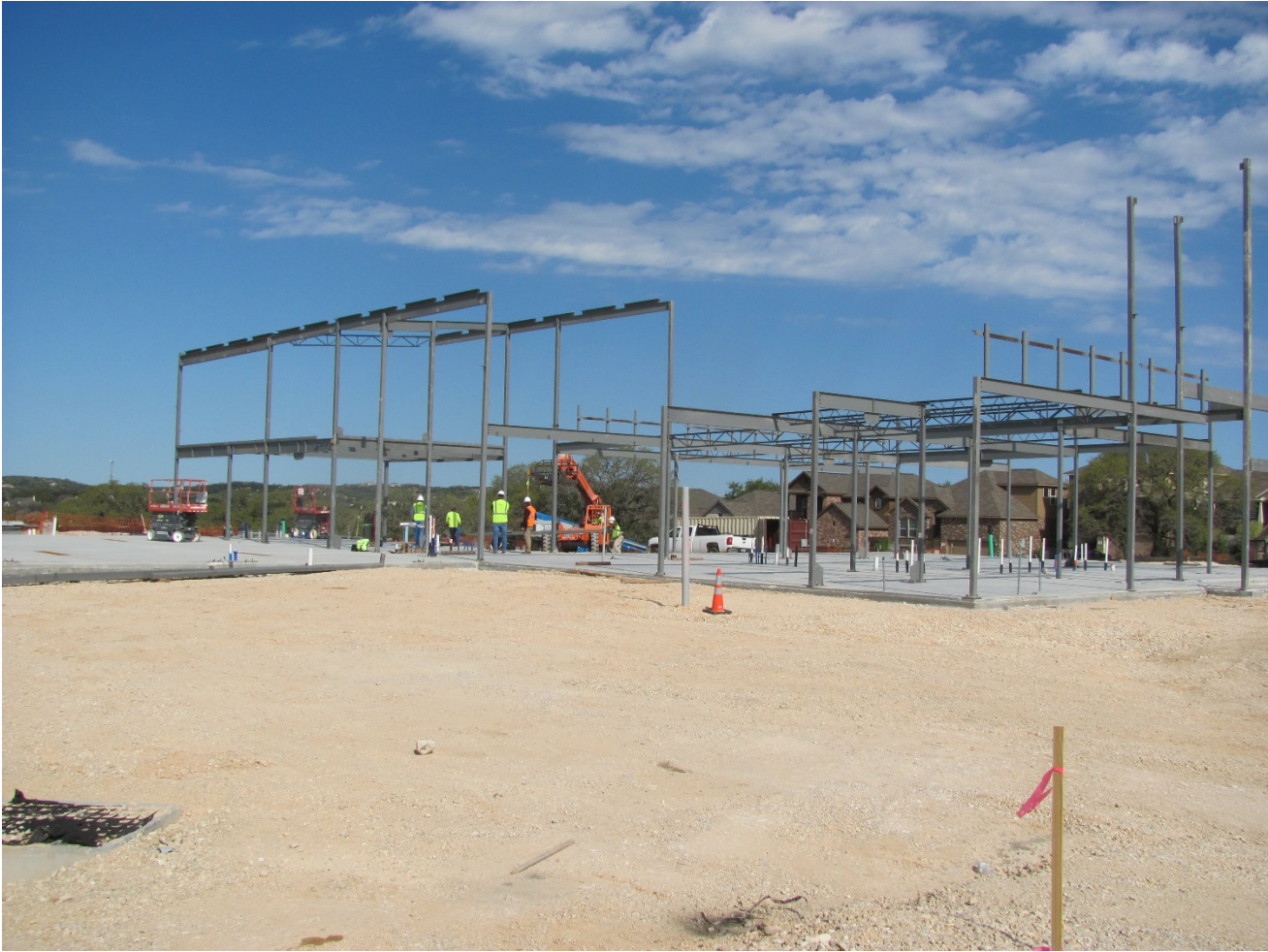
EXHIBIT 6 – STRUCTURAL STEEL ERECTION – WORKING DAY 5 03.29.21
