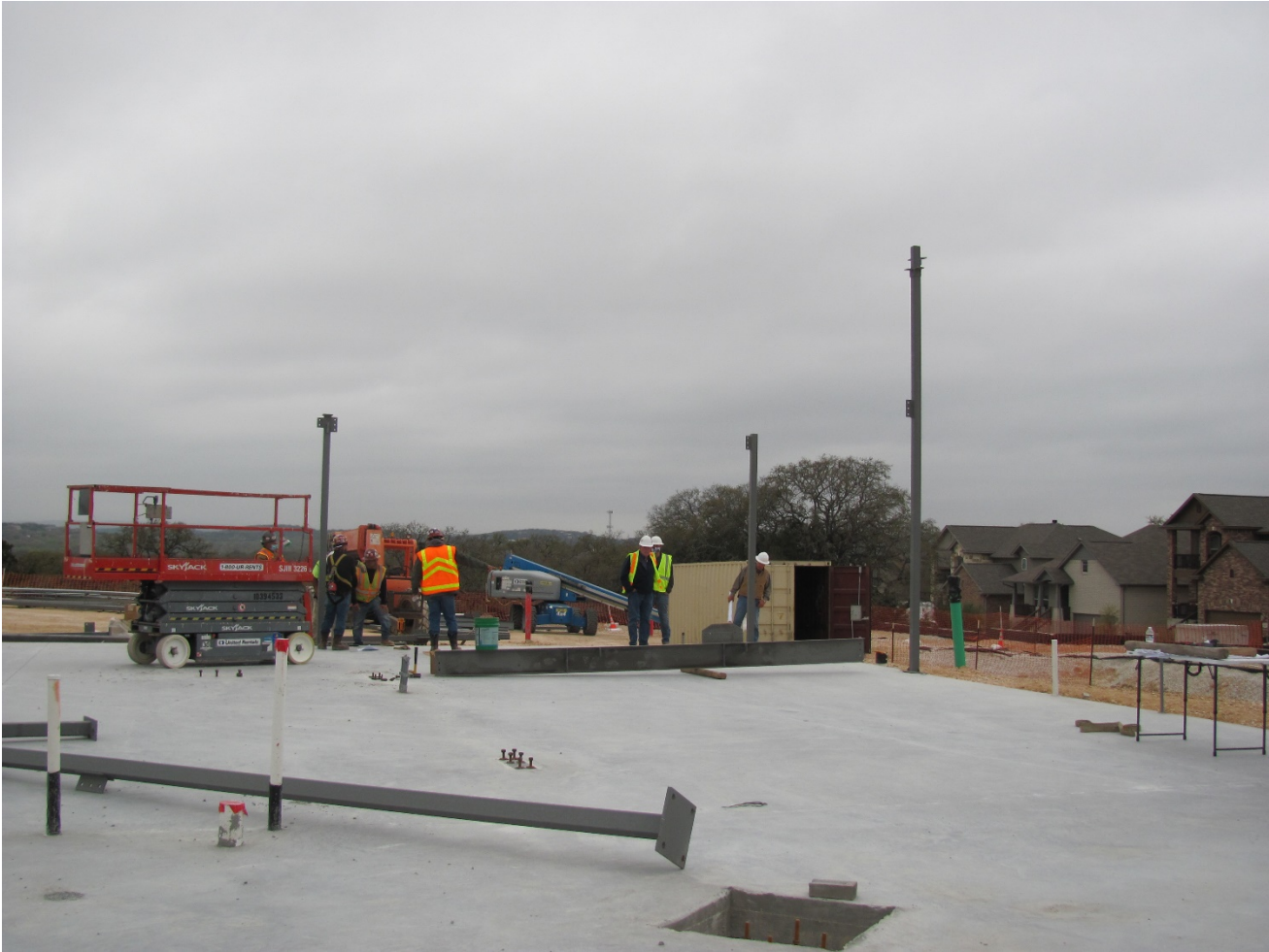
EXHIBIT 3 – START STRUCTURAL STEEL ERECTION – WORKING DAY 1 03.23.21
