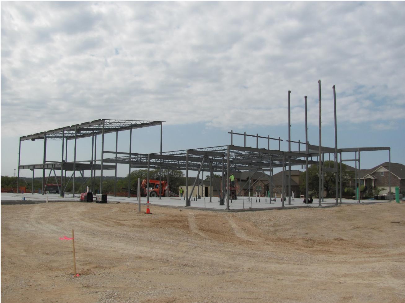
EXHIBIT 7 – STRUTURAL STEEL ERECTION – WORKING DAY 5 03.29.21
