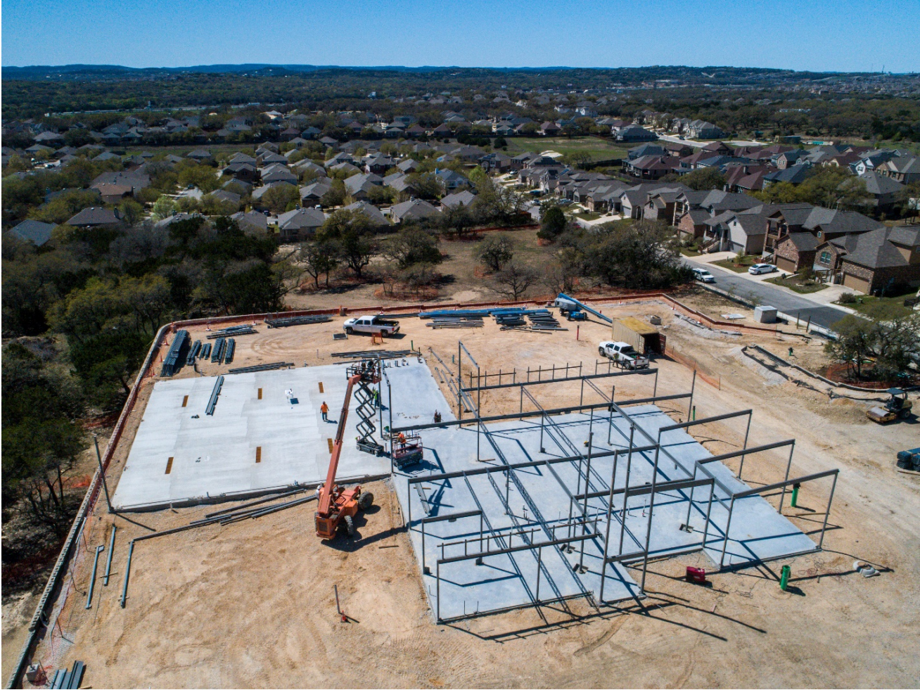
EXHIBIT 5 – STRUCTURAL STEEL ERECTION – WORKING DAY 3 03.25.21
