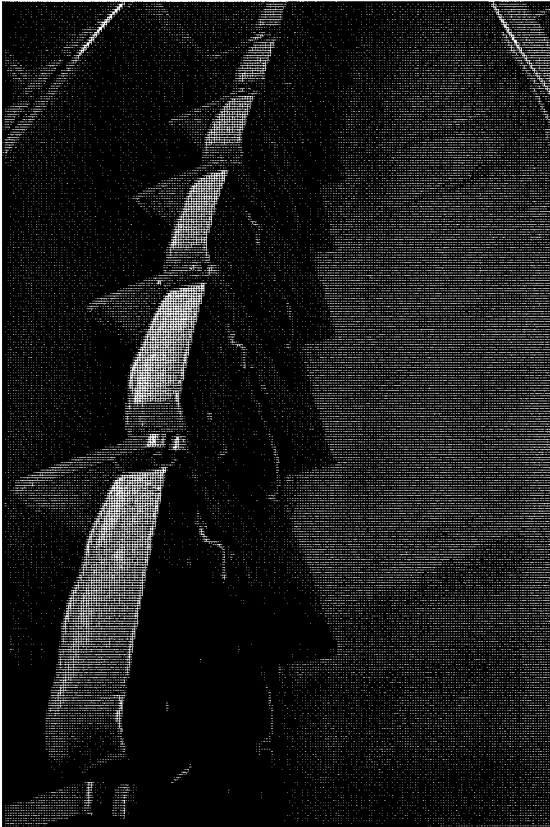
Fig. 33: Auditorium; Original fold down theater-type seats, with metal hat holders on the underside
