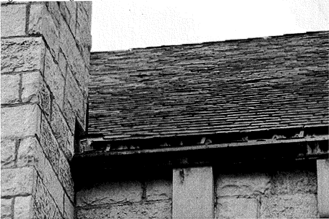
Fig. 1: Slated Shingle Roof, West side
