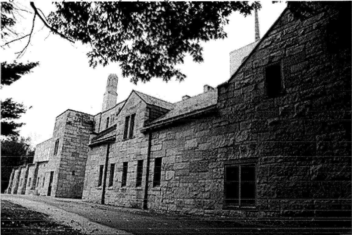
Fig. 2: West Facade, driveway to parking lot
