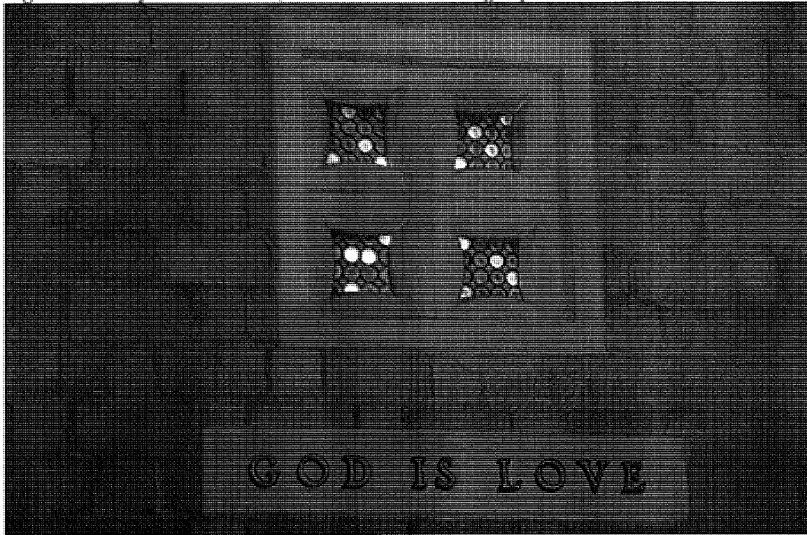
Fig. 59: Sunday School Room, West Wall above stage space
