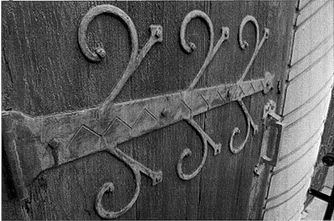
Fig. 9: North door, metal strap work
