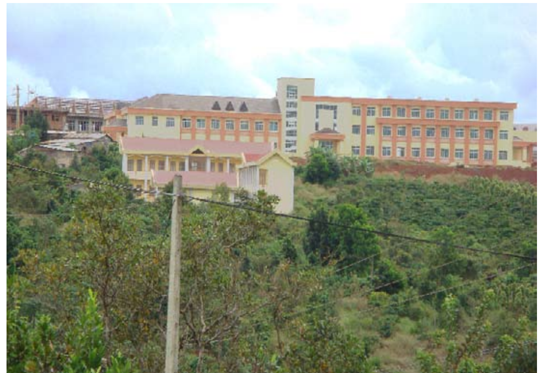
fig.12 Below Hospital Now under construction
