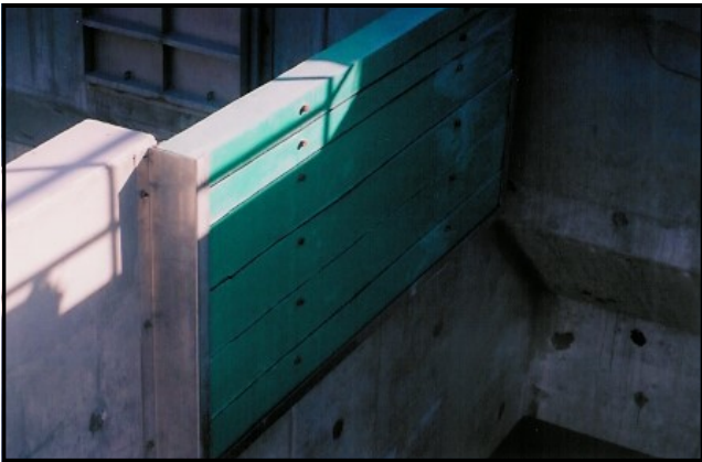
Las Vegas, NV Type "B" Stop Logs 10'0" clear span rated for 8' of head
