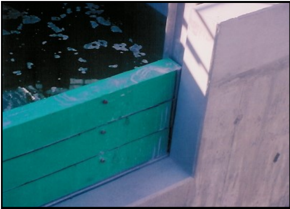
Las Vegas, NV Type "B" Stop Logs 10'0" clear span rated for 8' of head
