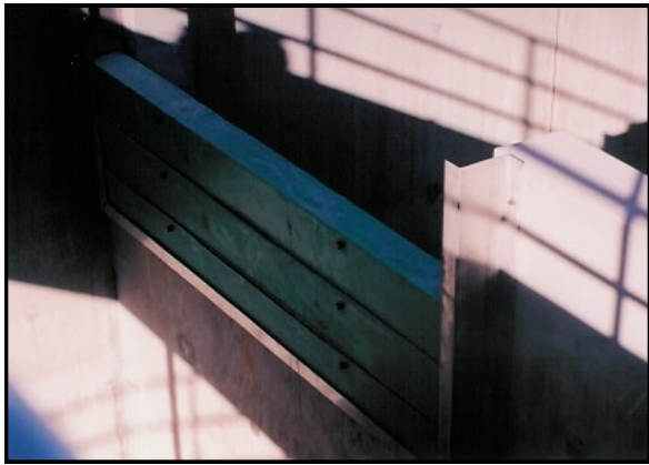
Las Vegas, NV Type "B" Stop Logs 10'0" clear span rated for 8' of head
