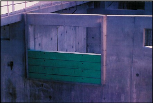
Las Vegas, NV Type "B" Stop Logs 10'0" clear span rated for 8' of head
