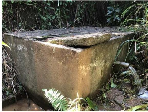
**Filter plugged and flowing improperly**
