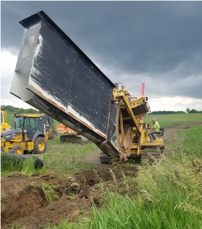
Above: Tile being installed to convey water from upstream tile outlets and a road culvert– Below: Water going into the newly installed tile intake shortly after construction
