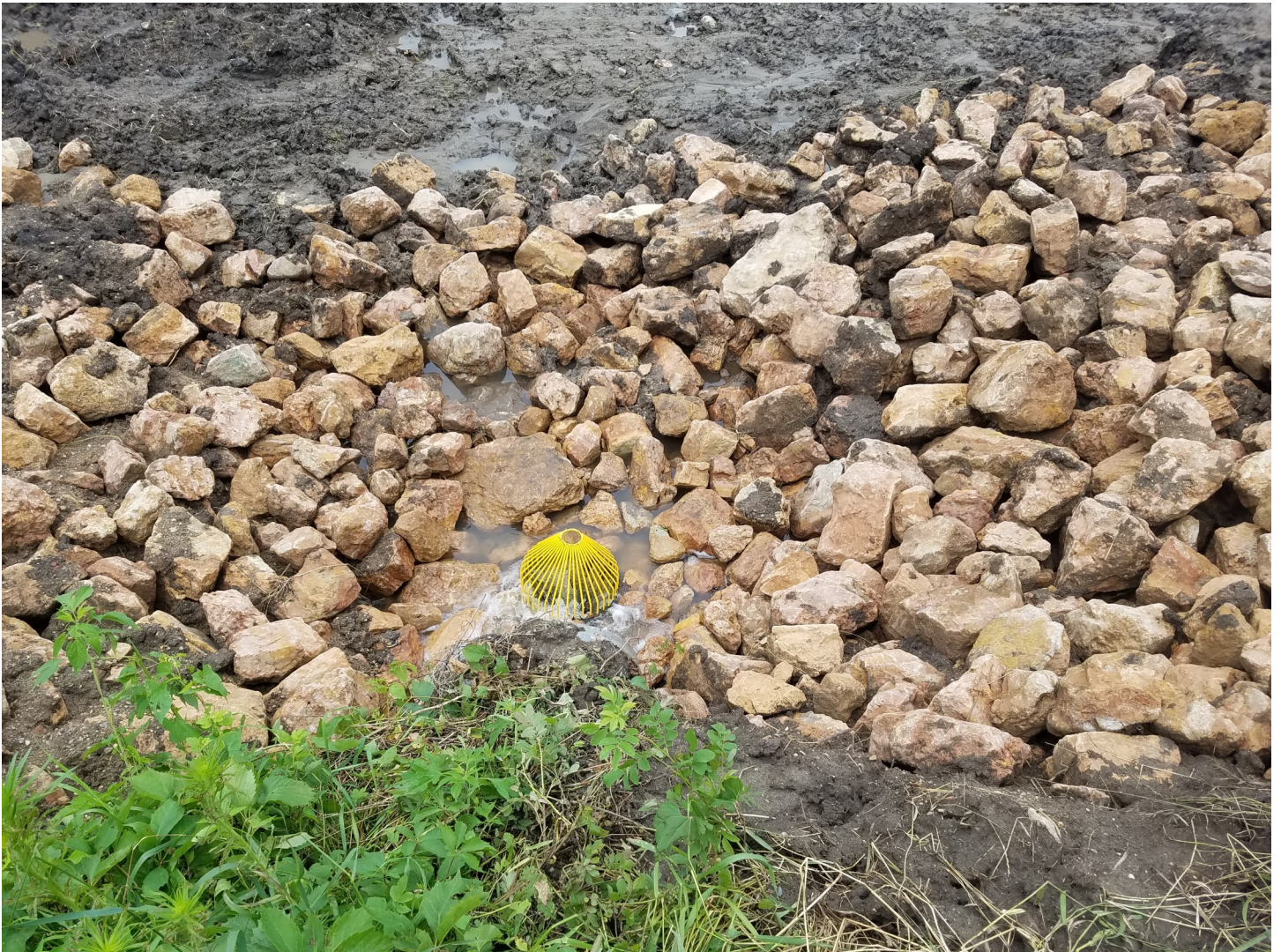
Above: Tile being installed to convey water from upstream tile outlets and a road culvert– Below: Water going into the newly installed tile intake shortly after construction
