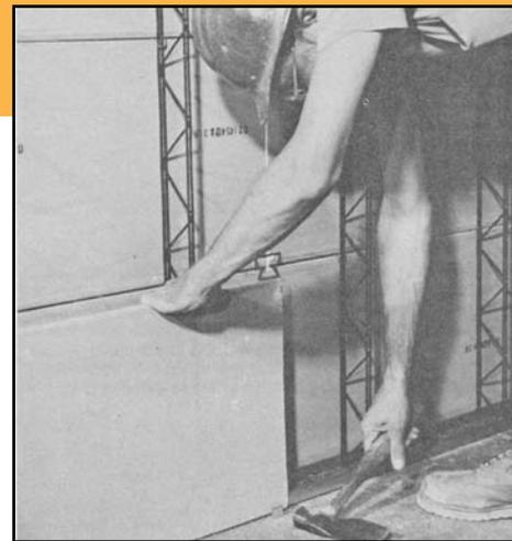
*Before the advent of the self-drilling screw, attachment of sheathing to steel framing was difficult and time consuming. Special clips were developed for some applications, after attempts to develop a nailable stud were unsuccessful.*
