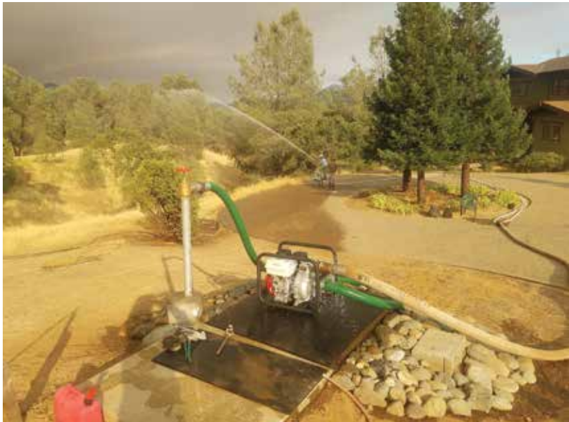
LEFT: A gas-powered fire pump effectively increases the water pressure of a domestic water service into powerful fire hydrant pressure. It pulls water from the McGanns' 10,000-gallon concrete water tank. With this system, the McGanns were able to begin defending their home. RIGHT: The McGanns store their portable gas-powered fire pump and auction-bought used fire hose in their "fire pump station."
