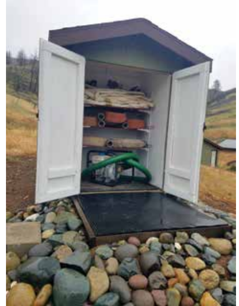
LEFT: A gas-powered fire pump effectively increases the water pressure of a domestic water service into powerful fire hydrant pressure. It pulls water from the McGanns' 10,000-gallon concrete water tank. With this system, the McGanns were able to begin defending their home. RIGHT: The McGanns store their portable gas-powered fire pump and auction-bought used fire hose in their "fire pump station."
