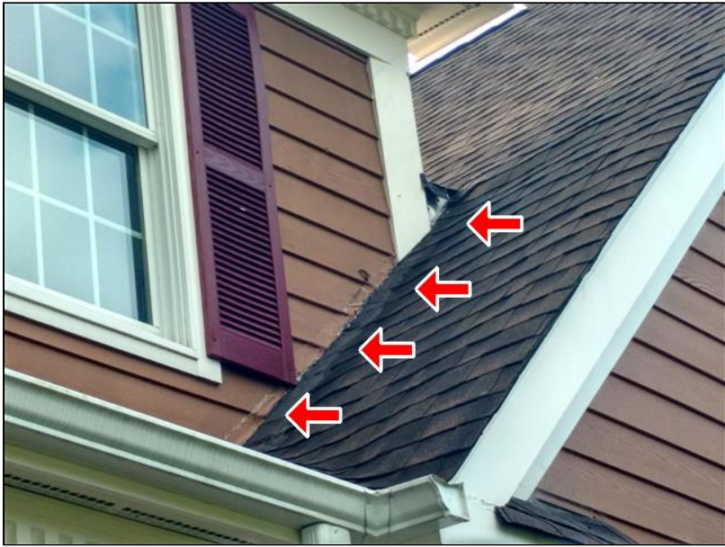
2.0 Item 15 (Picture) Sub standard repair
