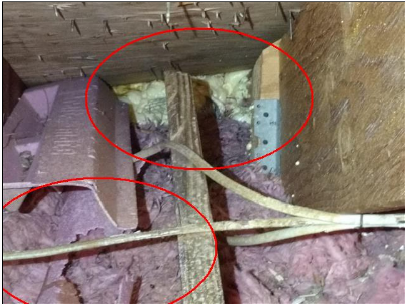
6.0 Item 9 (Picture) Baffles damaged
