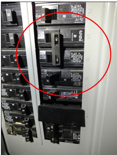
14.9 Item 3 (Picture) Circuit breaker off
