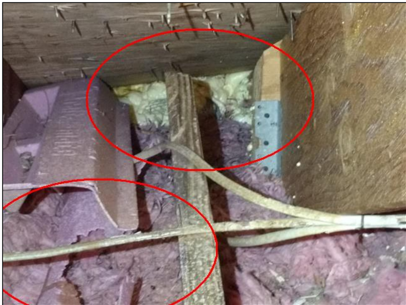
6.0 Item 9 (Picture) Baffles damaged
