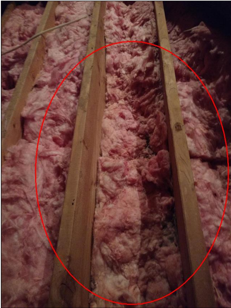
6.0 Item 3 (Picture) Damaged insulation
