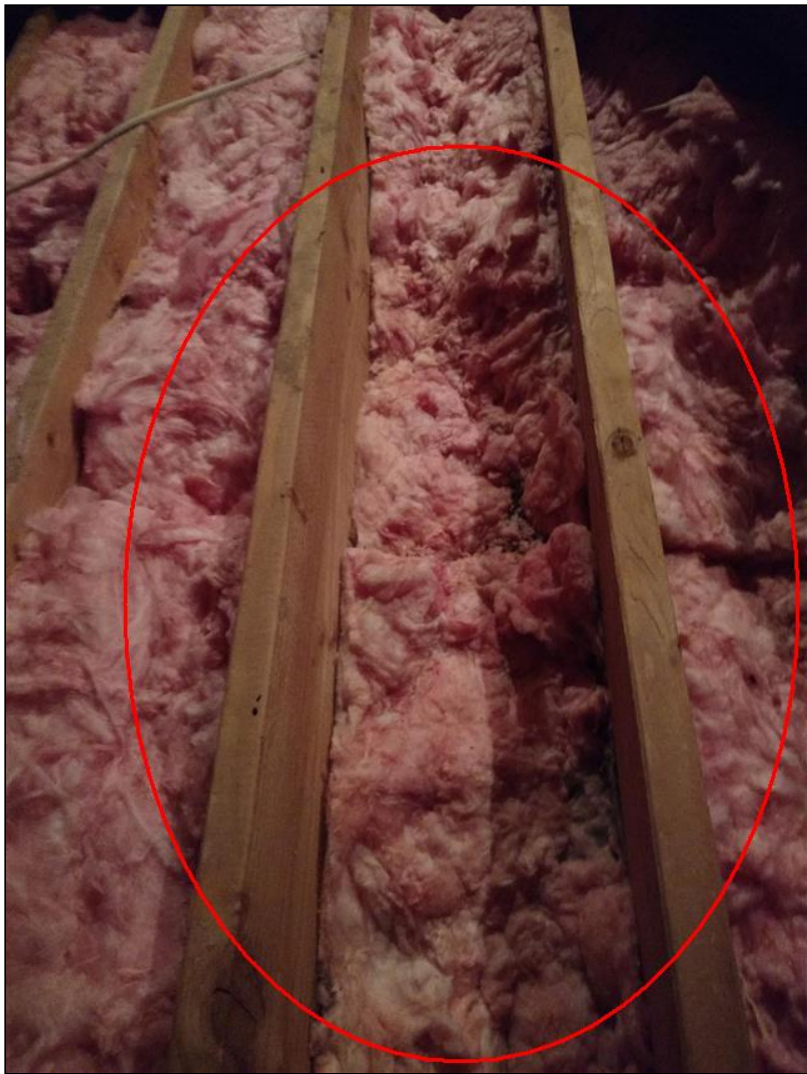
6.0 Item 3 (Picture) Damaged insulation
