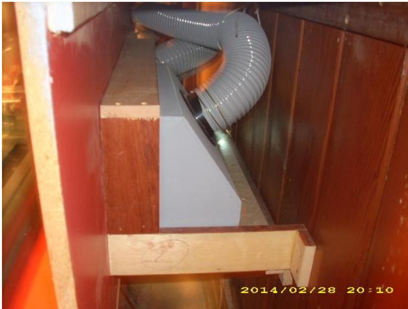
Two 4" diameter flex hoses connect the ports in back of the collector boxes to a common connector for the cyclone dust collector.
