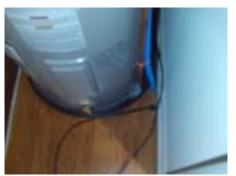
The pressure relief valve is leaking.
