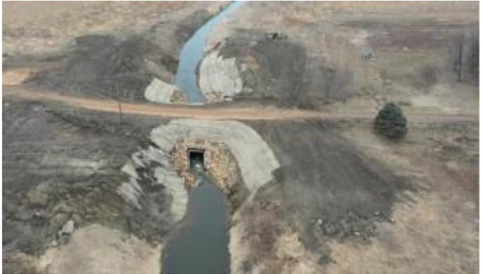
*JD54 Box culvert replacement from the flooding of 2019 located in Lanesburgh Township.*
