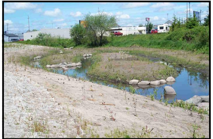
Amazon Creek upstream, near Oak Patch Road. This section was recently widened and could be similar to the channel treatment near Dragonfly Bend. Photo above was taken shortly after channel widening.
