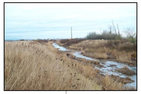
Reservoir via the Amazon Diversion Channel, which was constructed by the Corps in the mid-1950s. In 1965, the SCS proposed a watershed plan for lower Amazon Creek. Under this plan, Amazon Creek, between the Diversion Channel and Clear Lake. was further channelized and cleared of woody vegetation to improve flow. A relatively low levee (spoils from deepening) lines each side of the channel and is between one and two feet higher than the grade of the adjacent field (See cross
