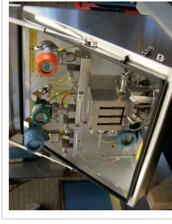
High integrity manifold block with key interlock system
