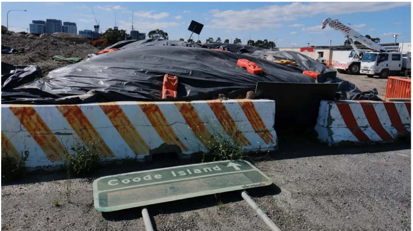
PFAS-contaminated soil from the West Gate Tunnel is being stored in west Melbourne while the government and contractors try to find permanent disposal sites. Luis Enrique Ascui
