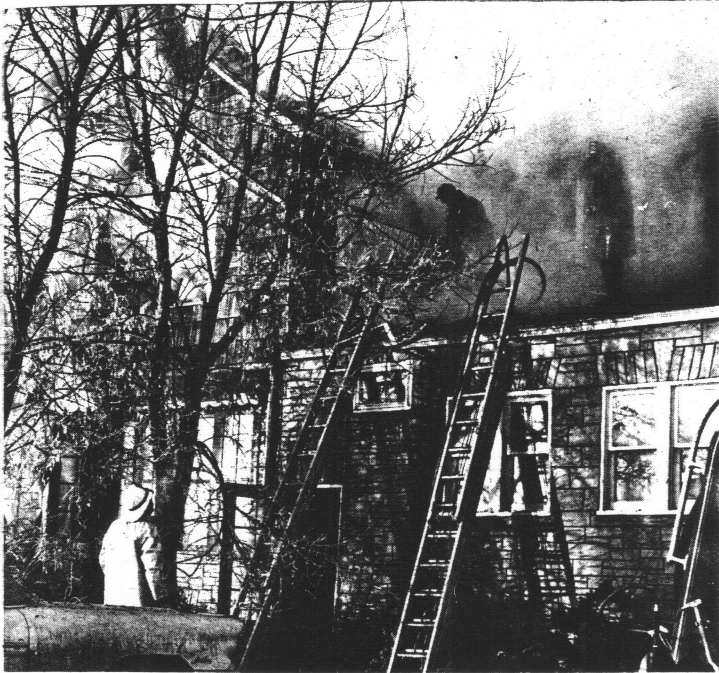
THE RESIDENTIAL portion of the Y Bowl on Racine ave. in Muskego was badly damaged by a fire in near-zero weather Saturday afternoon. Muskego firemen were assisted by units from Tess Corners, Big Bend and New Berlin. Another photo is on page two of this issue. (Hub photo)
