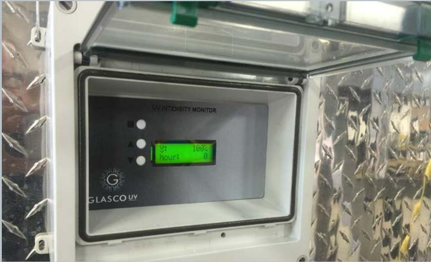
UV Monitor is contained in a remote NEMA 4x fiberglass enclosure with gasketed seals. Enclosure has a port to access the 4-20 mA signal.
