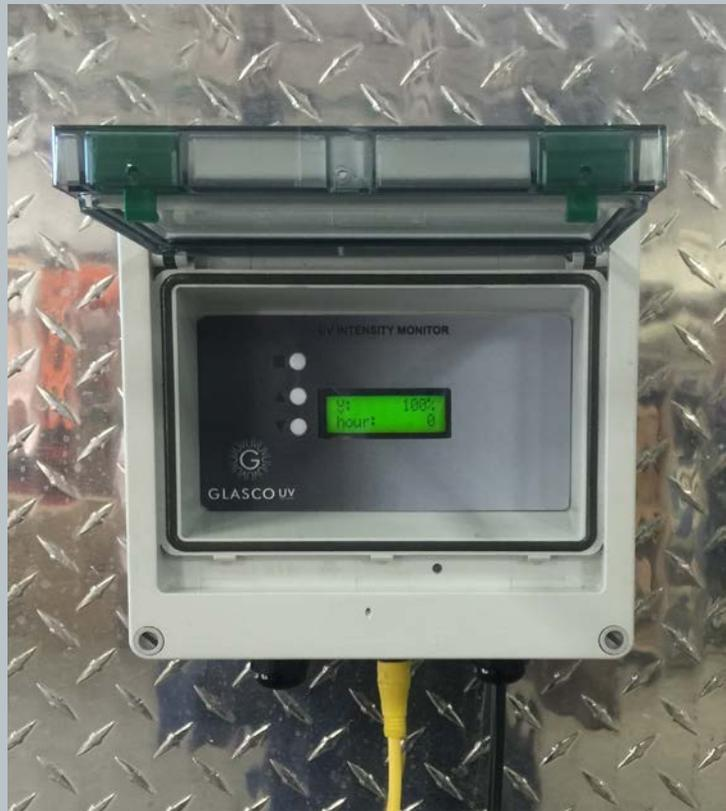
UV meter is field adjustable and can be re-calibrated when new lamps are installed.
