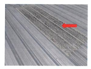
There are 13 skylights located on building 1. These are a clear plastic, fiberglass reinforced panel. The skylights are deteriorating and becoming more brittle. As the skylight deteriorates more, it will start to crack and leak at the fasteners. This can cause roof leaks and structurally weaken the skylight. This is then a vulnerable opening in the roof.
