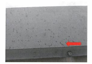
The coated metal has areas where the factory paint has blemishes and is deteriorating. This is where initial surface rust will start to show from the metal not being protected.
