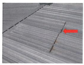
Typically the first places that see rust are along all the rough cut panel edges. The metal panels are coated with a clear acrylic coating. When the panel is cut, this leaves an unprotected edge. This edge is where the first signs of rust will begin.
