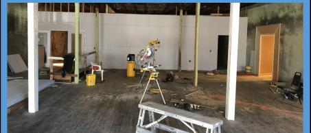
Drywall has been installed. This is a view from the front doors looking into the new visitor center. The double door on the left side leads into the boardroom. The door on the right side leads into the foundation and magazine offices. The entry on the right leads into the art center and public restrooms. The tin ceiling in this room will be 10 feet tall and the columns will be wrapped.
