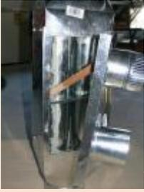
12. With it pop riveted together or sheet metal screws, this is when i used the duct sealant over any possible leakage area. After that was done I bent the flat sheet metal around the register ducts, fastening with sheet metal screws as I went along.
