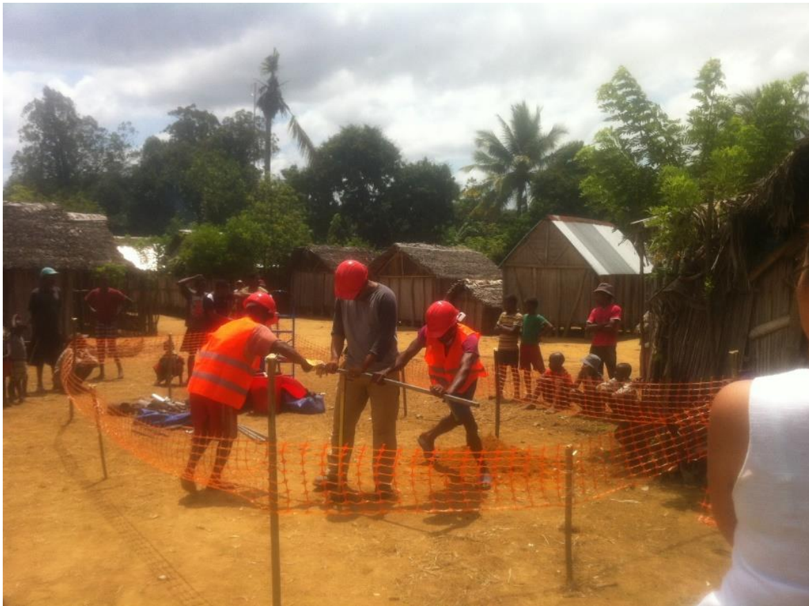
Drilling Operations in Ambodivaro
