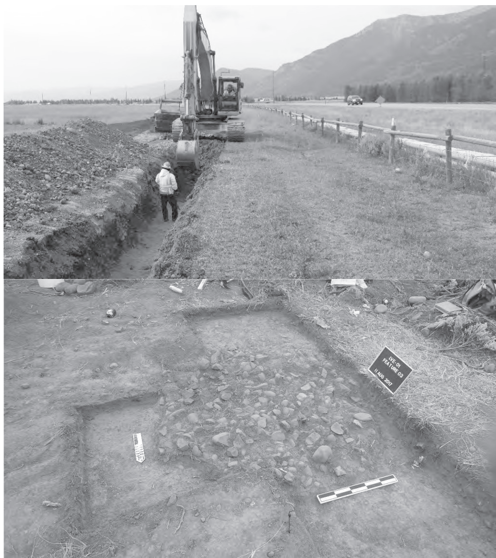
Feature 3, 48TE2027 facing southwest (dated to 1430 ± 25 yrs BP). Photographs courtesy of Cannon Heritage Consultants, Inc., Logan Utah.
