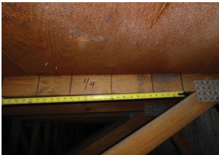
#3 ROOF DECK ATTACHMENT 6" X 6" NAIL SPACING
