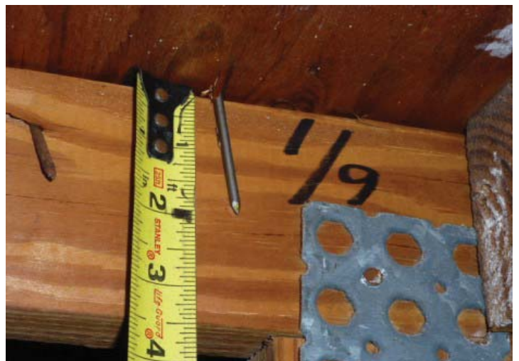
#3 ROOF DECK ATTACHMENT 8d NAILS
