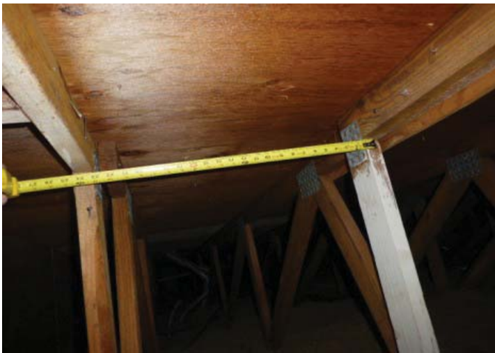
TRUSS/RAFTER SPACING
