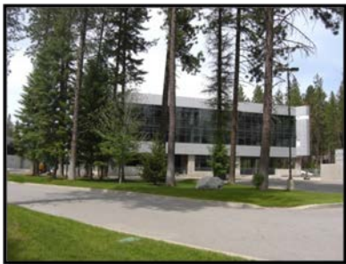
Coldwater Creek Center
