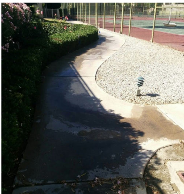
A lot of overspray from the hedges. These should also be watered with drip tubing.
