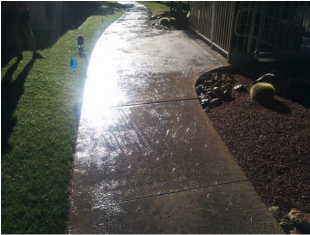
Overspray, not just onto sidewalk, but also into desertscape. This isn't good for either.
