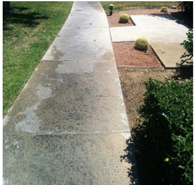
Should be drip, instead of sprinklers here.
