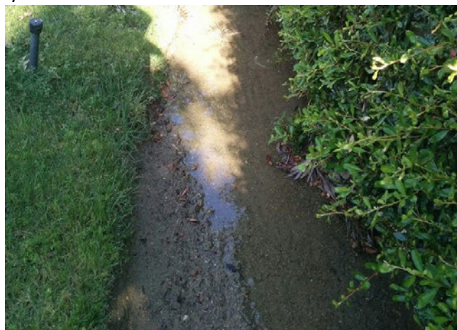
Flooding from blocked spray heads, another opportunity for drip tubing
