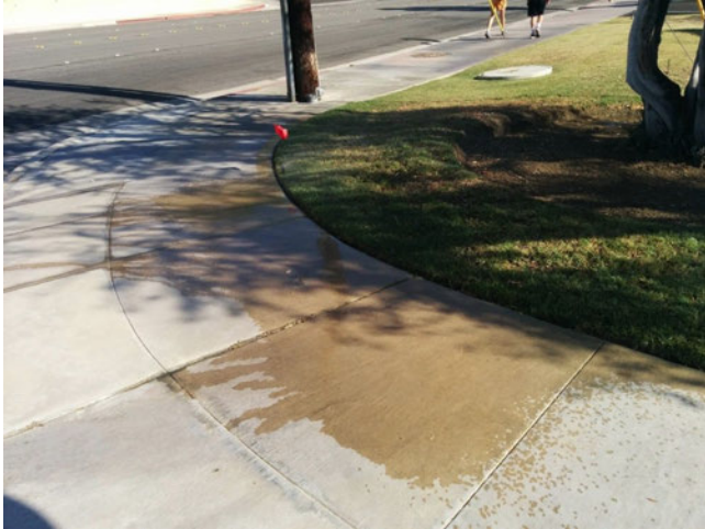
Overspray onto sidewalk
