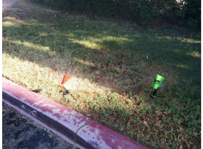
Poor (redundant) sprinkler placement
