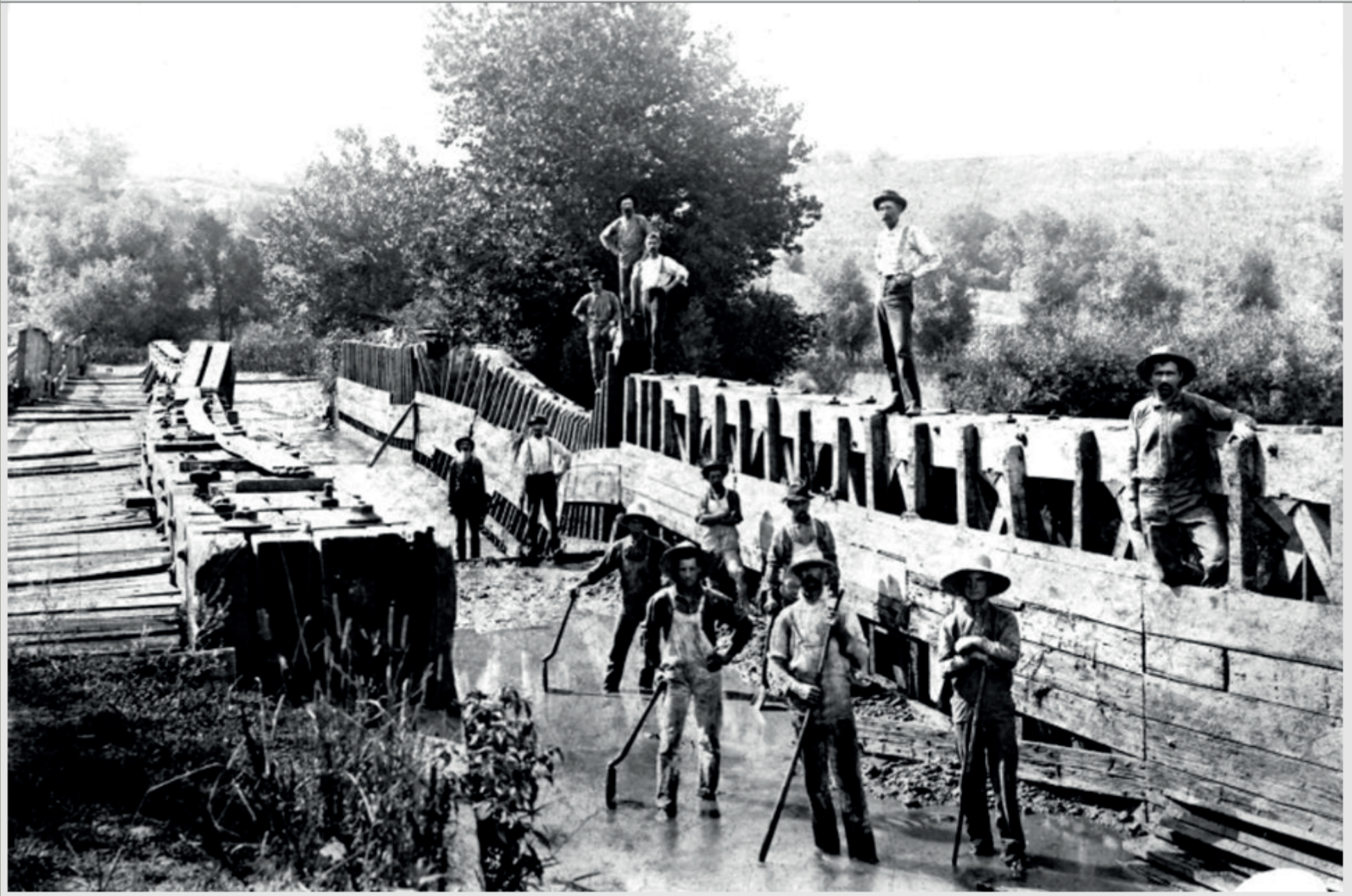
O & E Walhonding Aqueduct Repair crew ca 1880s Photo credit Univ of Akron Louis Baus collection
