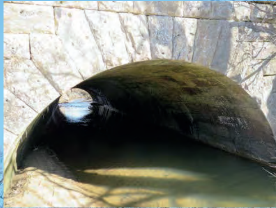
Crooked Run Culvert RR side circa 1890s. 2018
