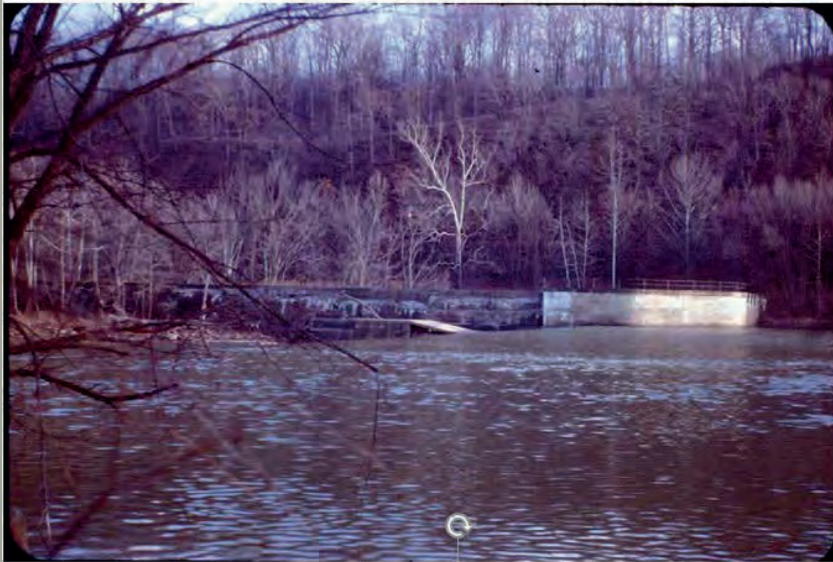
Walhonding 6-Mile Dam . Jan 1965. Per Terry Woods: "This photo was taken probably from a boat, just above the dam looking downstream. The gray structure to the right and extending to the left of the photo is the concrete protection wall erected in 1909 after the previous earthen protection embankment was swept away in high water. The entrance to the old Hydro Race is between the dark and light concrete. You can see the crest of the dam in the photo. The canal was still watered down to Hosfelt's Wasteway when this photo was taken. Lock 4 (a guard lock) is about 3/8 of a mile downstream from this point. (Photo credit: Unknown).
