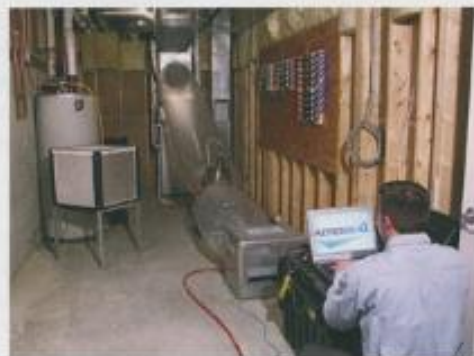
Inside job. AeroSeal uses a process in which a nontoxic mist is sprayed inside the home's ductwork system. The company says that the aerosol finds and seals even the most inaccessible leaks.
