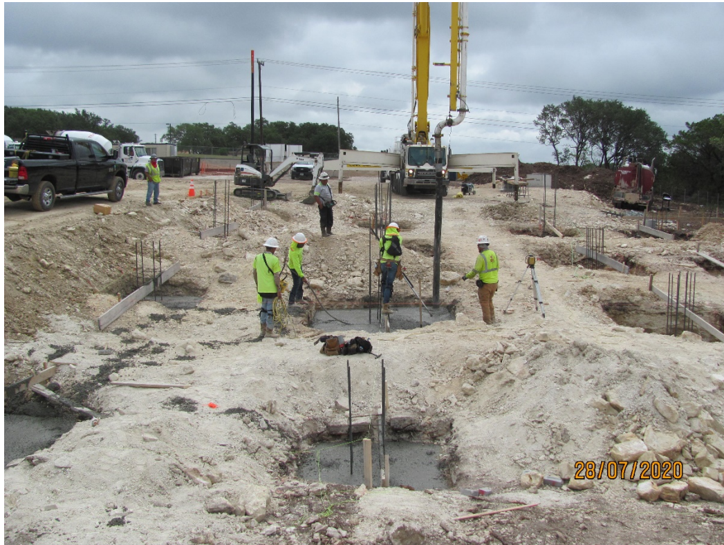
EXHIBIT 11 – CONCRETE POUR FOR SPREAD FOOTINGS 07.28.20
