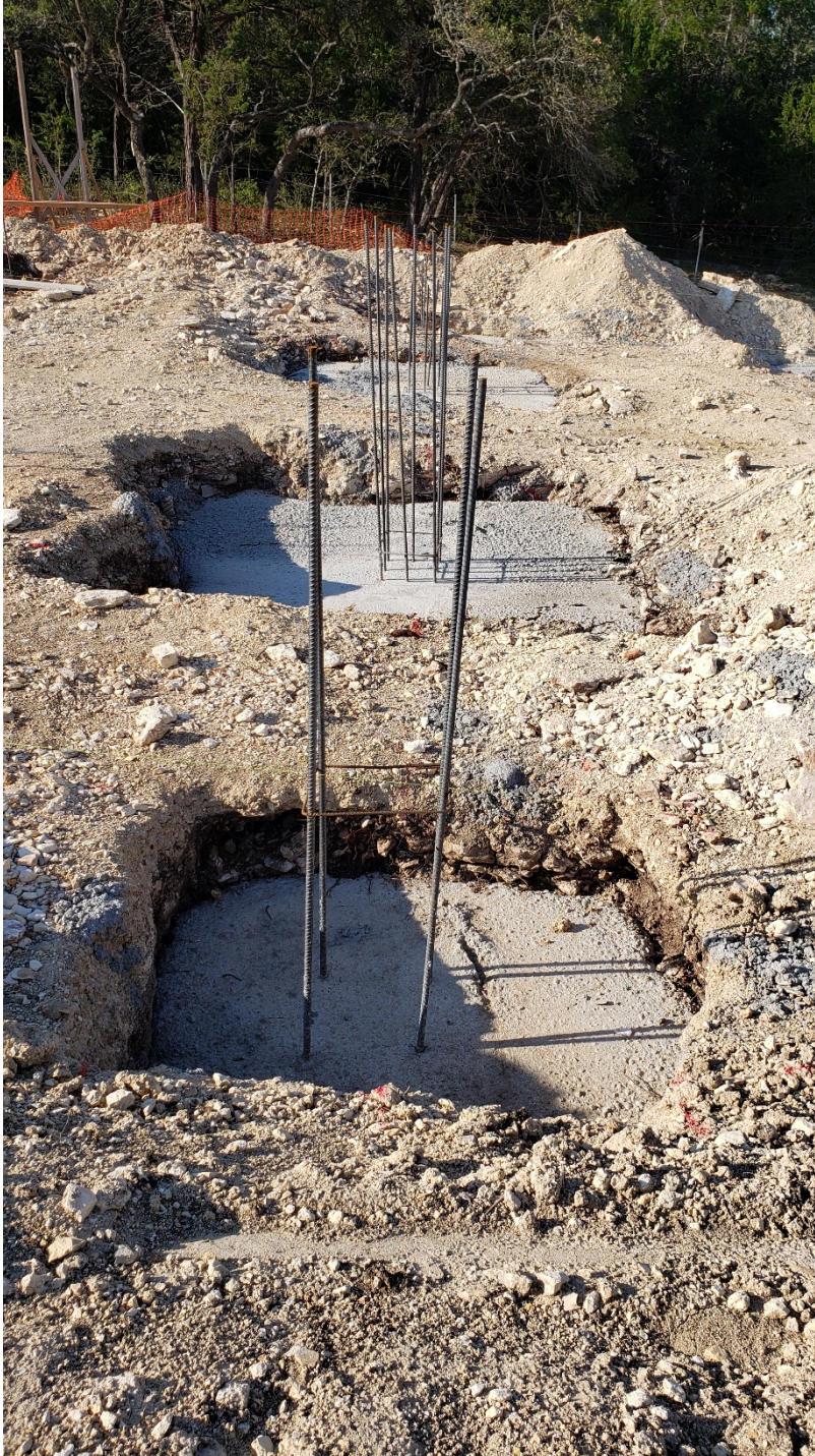
EXHIBIT 14 – CONCRETE SPREAD FOOTINGS FOR CONCRETE COLUMNS
