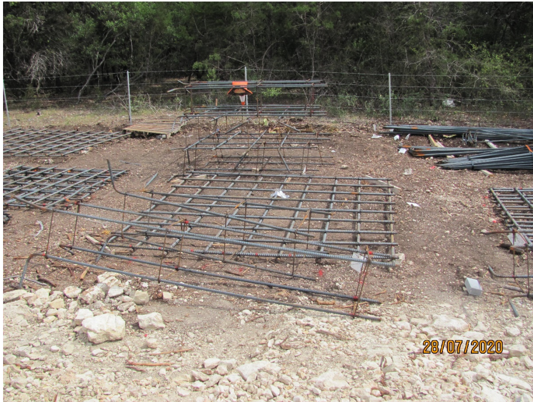
EXHIBIT 9 – REBAR REINFORCEMENT FOR SPREAD FOOTINGS 07.28.20
