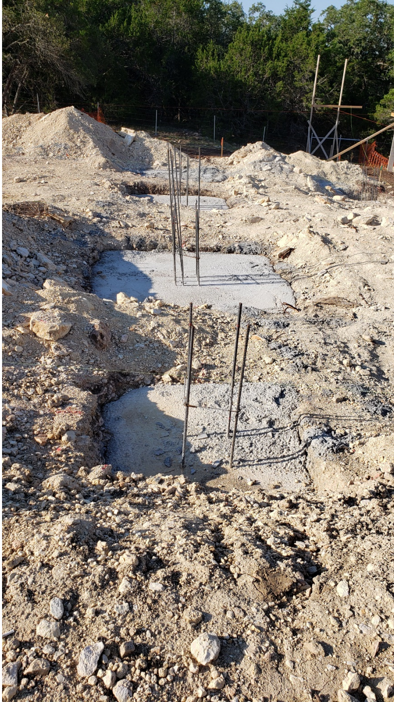
EXHIBIT 13 – CONCRETE SPREAD FOOTINGS FOR CONCRETE COLUMNS
