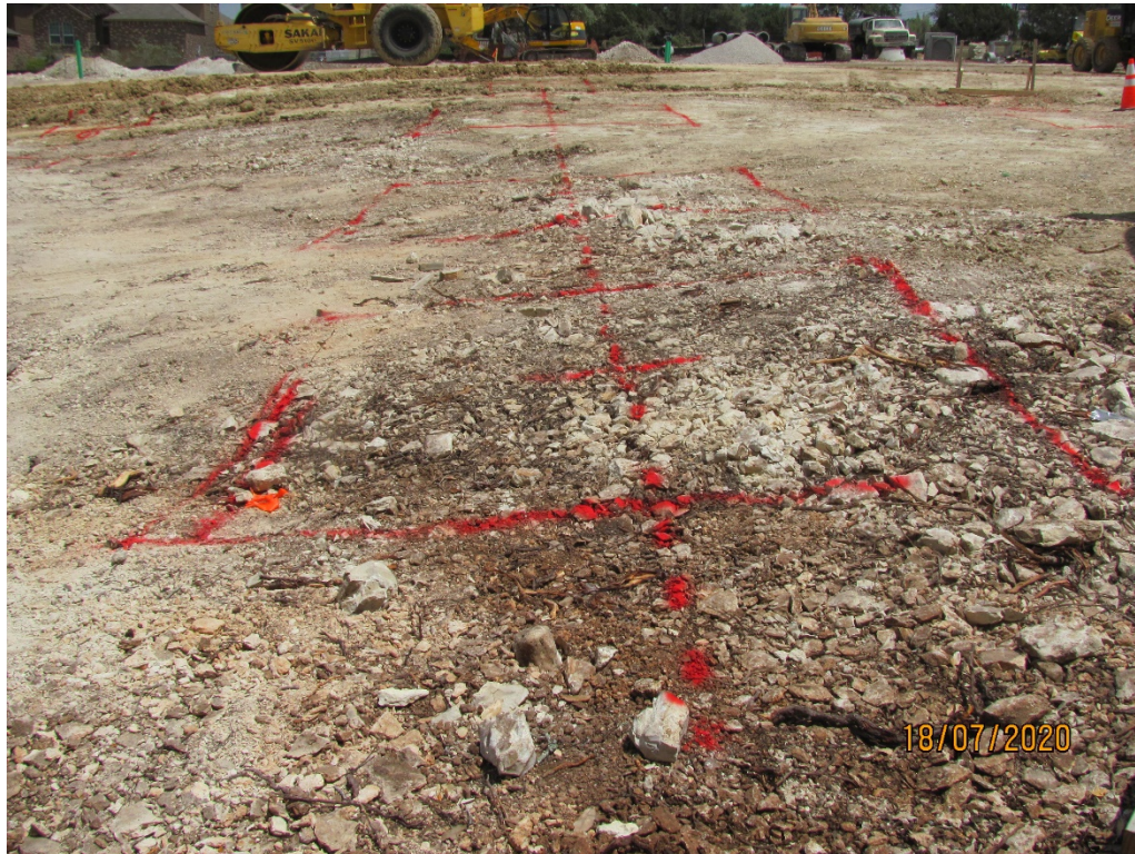
EXHIBIT 7 – GRID LINES / MARKS FOR SPREAD FOOTINGS 07.18.20
