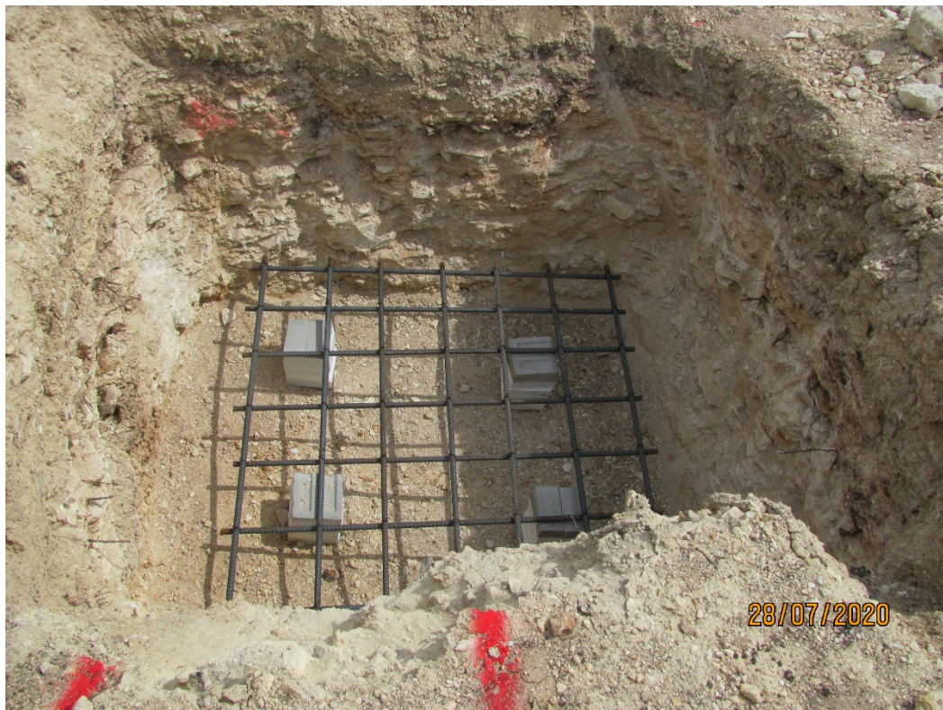
EXHIBIT 10 – REBAR FOR SPREAD FOOTINGS IN EXCAVATED PIT 07.28.20
