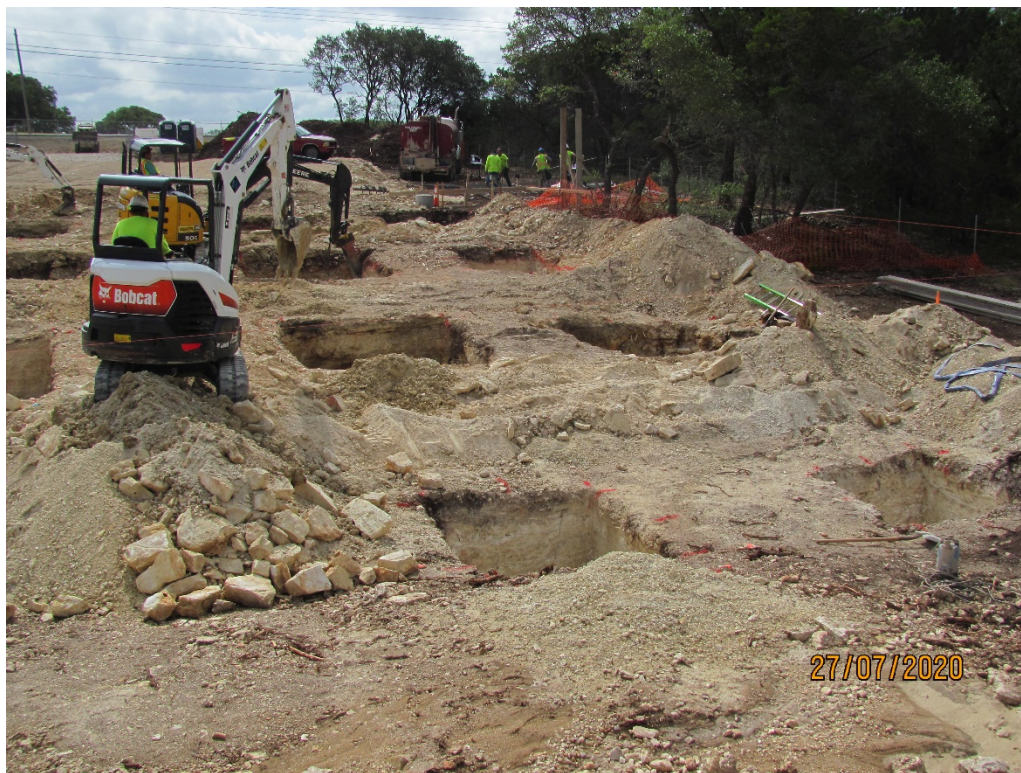
EXHIBIT 8 – EXCAVATION PITS FOR CONCRETE SPREAD FOOTINGS 07.27.20
