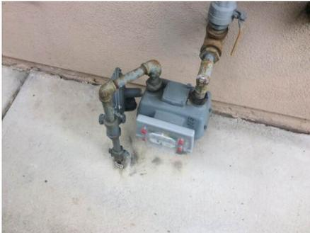
• There is no wrench at the gas shut-off valve to facilitate an emergency shut-off, and inasmuch as such tools are relatively inexpensive we recommend that you buy one and leave it in-place on the valve
