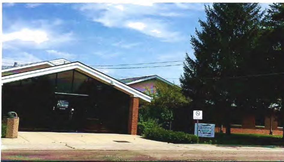
Addictions Recover Center building at 498 NW 18th St. Building 416 Richmond, IN 47374
